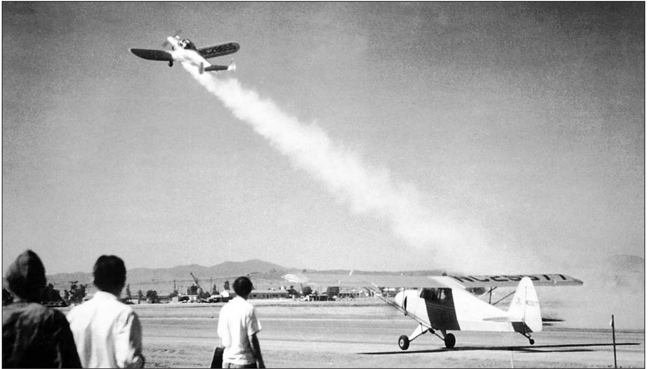
*The United States' first rocket-assisted airplane takes off on August 12, 1941. The Ercoupe plane was fitted with a solid-propellant 28-pound-thrust JATO (jet-assisted takeoff) booster. (NASA)*
