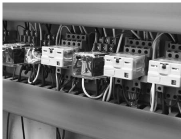
Fig. 1 Relay logic to cycle certain zones, temporarily, with timed-out latch release.
