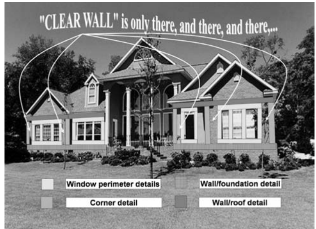
Fig. 3 Framing lies behind a significant portion of the wall area in many houses.
