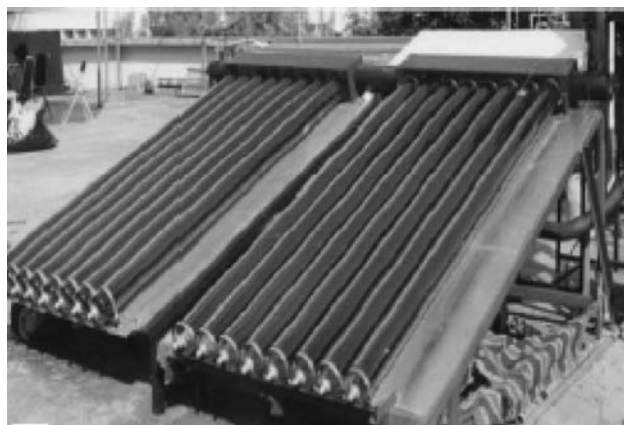
Fig. 5 Evacuated heat pipe collectors. Source: From Elsevier (see Ref. 8).
