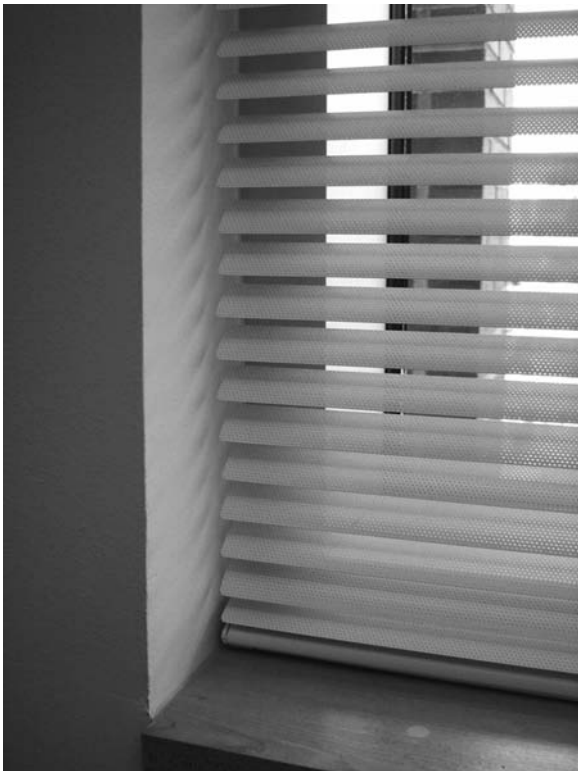
Fig. 2 Venetian Blinds: typical example of the manually controlled interior shading devices. The slats are made of perforated aluminum.
