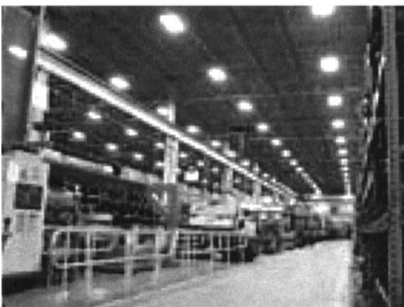
Fig. 6 Fifty percent more light obtained through lighting retrofits in a warehouse.
