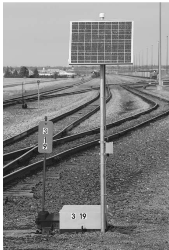
Fig. 10 A photovoltaic (PV)-powered rail yard switch near Alliance, Nebraska (Photo by Susan Ropp).
