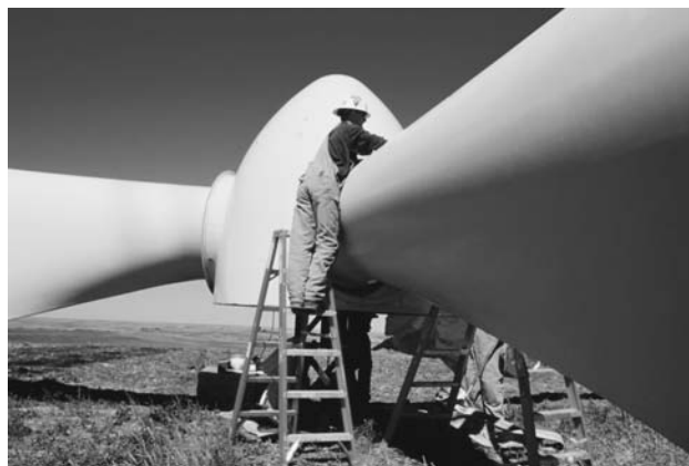
Fig. 2 Site assembly of large wind turbine nacelles and blades. (Photo courtesy of Suncor Energy, Inc.)
