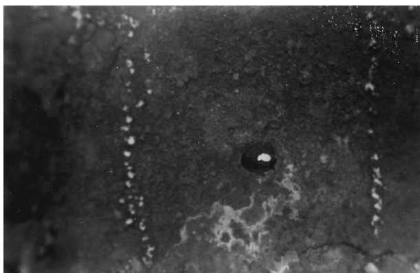
FIGURE 2.4 Close-up view of the leaky hole on the cut sample, as seen on the inside surface. Initiation of the hole on the inside surface and growth towards the outside surface can be seen.
