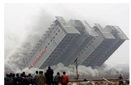
Dustin Broadbery: The Controlled Demolition of Society viewed recently: 2440
