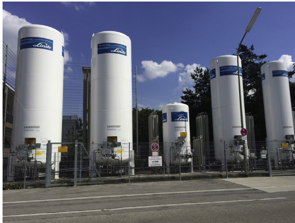
Figure 4.29 Central gas supply of a modern hospital with an easy to reach channel of supply for big trucks. From MITI.
