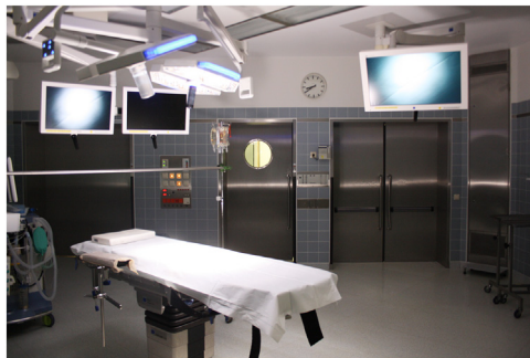
Figure 7.24 Monitors for laparoscopic surgery. Boom-mounted video screens can easily be positioned to provide “optical correctness.” The position of the surgeon, the working field, and the monitor have to be arranged in one line. From MITI.
