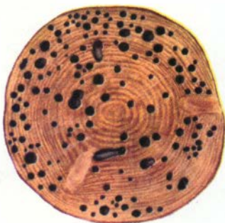
Damage to piling
