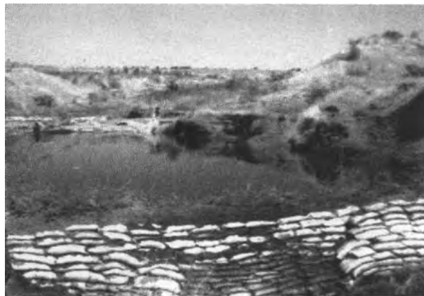
Fig. W.2: Excess run-off water is stored in shallow ponds for later use.
