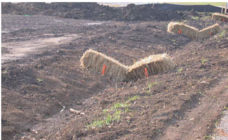
Fig. 11.24 Straw bales are used to stabilize waterways (Courtesy Ryan Bartels)
