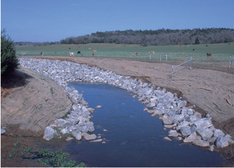
Fig. 11.2 Grade stabilization structures are established along drainageways to prevent gully erosion (Courtesy USDA-NRCS)
