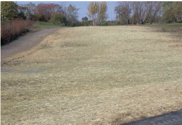
Fig. 12.11 Disturbed area seeded to grass under mulch cover (Courtesy Ryan Bartels)
