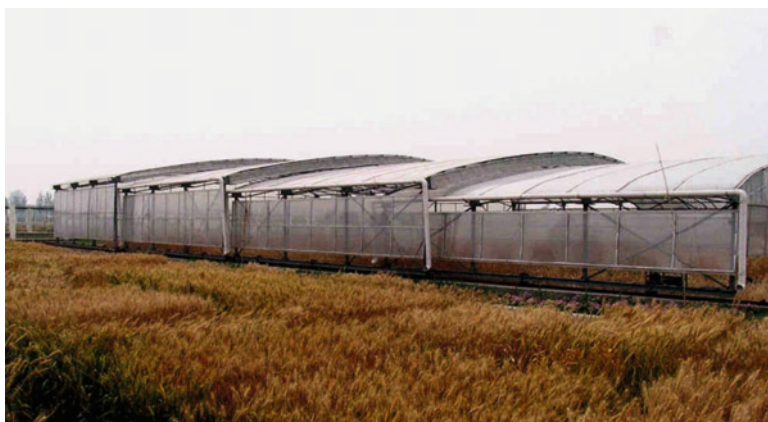
Fig. 4.5 Multi-cover installation combined of 4 roof sections set over the protected plot. Each section travels on its own tracks and sections are parked towards the far end one under the other when they are off the protected plot. Notice the water drains on each section (The Luoyang Station of the Luoyang Academy of Science, Henan China)
