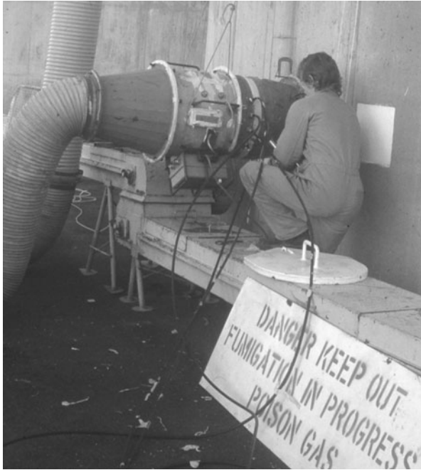
Fig. 10.4. Setting up for re-circulation fumigation of a vertical grain storage with methyl bromide, using an axial flow fan and heating to vaporize the gas before introduction to the base of the silo.
