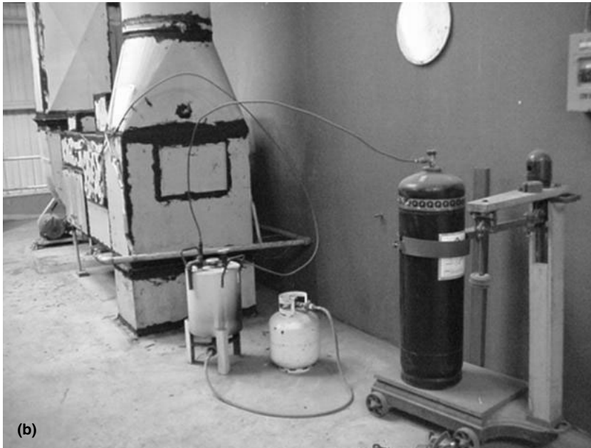
Fig. 10.2. Gassing equipment of a permanent fumigation chamber. (a) Note that the operator is using a positive-flow personal air supply as he controls the amount of gas admitted from the cylinder by weight using a heated vaporizer to ensure that the liquid methyl bromide is admitted as the gas phase. (b) A high volume extraction fan is installed to ensure rapid clearance of the gas after treatment is completed.
