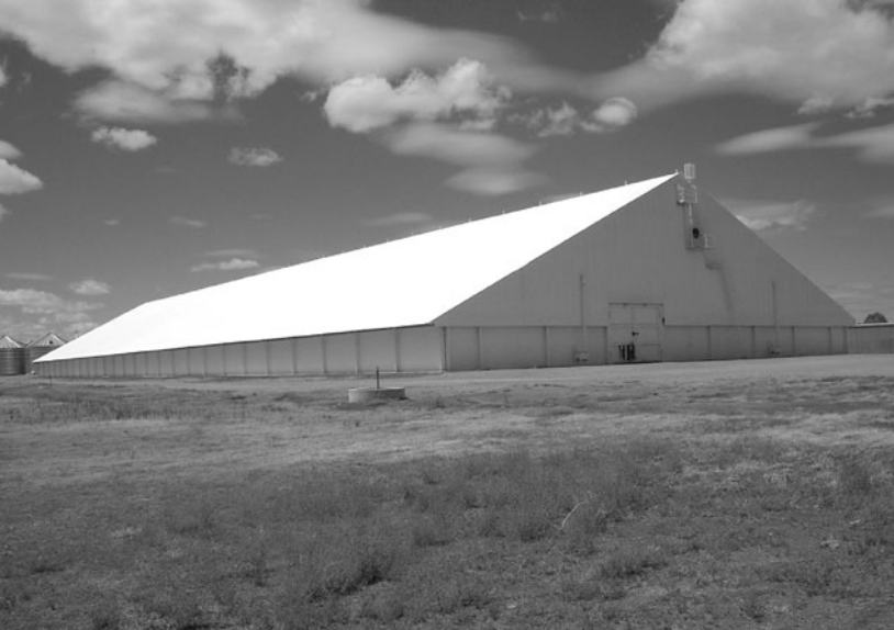
Fig. 11.1. An hermetically sealed grain storage with a capacity of 100,000 t (Moree, NSW, Australia) intended for modified atmosphere pest control. Structures of this size have low loss rates of the modified atmosphere because of their favourable surface to volume ratio.
