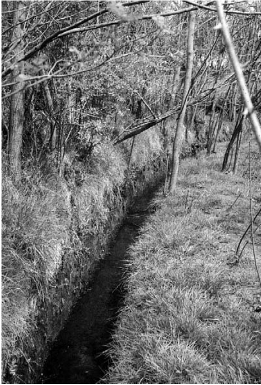
PHOTO 5.2. A narrow, active water channel showing uphill vegetative placement. This photo was taken in the winter before the leaves reestablished.
