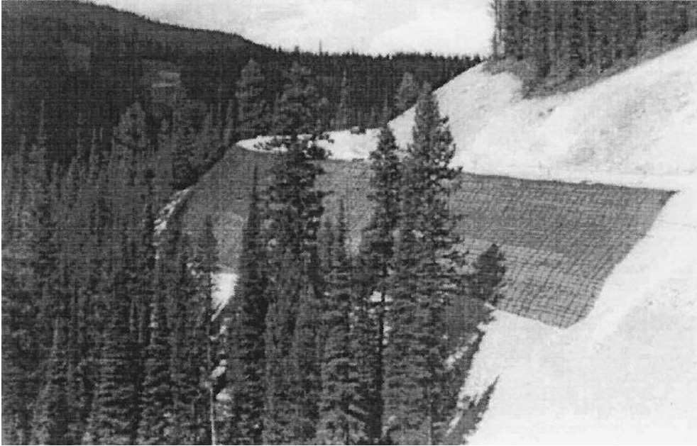
FIGURE 27.16 Erosion control mat placed to help establish the vegetation on the face of a 1H:1V reinforced soil slope.
