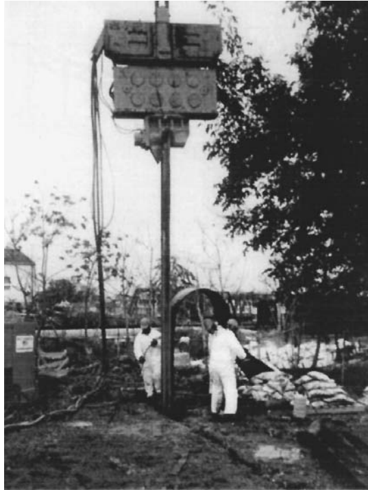
FIGURE 27.20 Installation of HDPE barrier wall utilizing conventional pile driving equipment. (Photo courtesy of Groundwater Control, Inc.)
