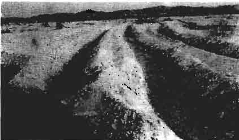
Figure 13.2.5. Spreading ditches in Tujunga Wash, Los Angeles, California (courtesy City of Los Angeles Department of Water and Power).
