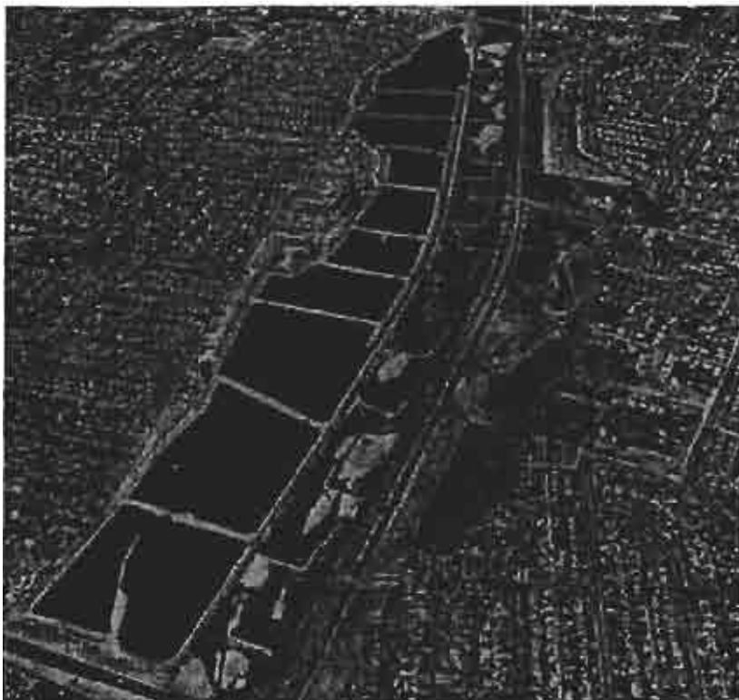
Figure 13.2.2. Aerial view of spreading basins adjoining the San Gabriel River, Los Angeles, California, and temporary finger dikes within the river channel (courtesy Los Angeles County Flood Control District).
