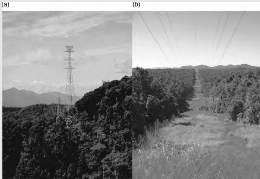
Figure 36.5 (a) The new Chalumbin–Woree powerline swings above the canopy between towers on ridge tops; (b) the grassland swathe of the Palmerston powerline clearing.
