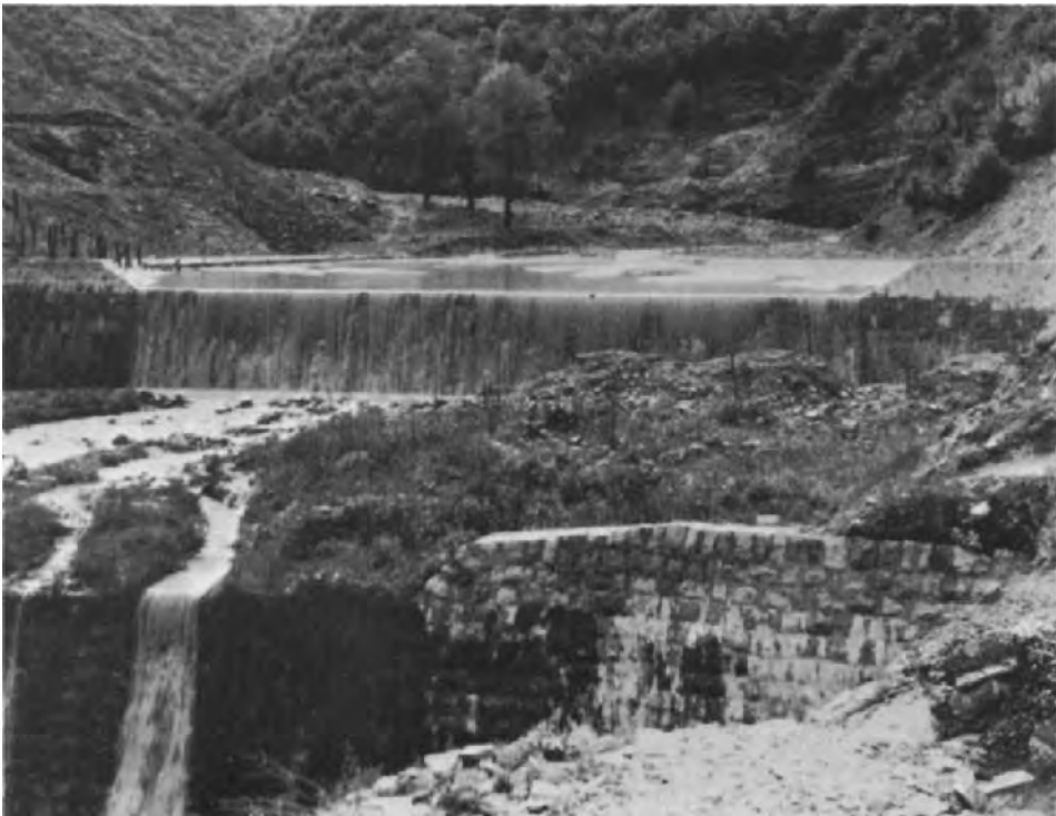
Fig. 149. Soil stabilization achieved with a flood retention barrier and forestation of the catchment area. (Photo D. Zachar.)
