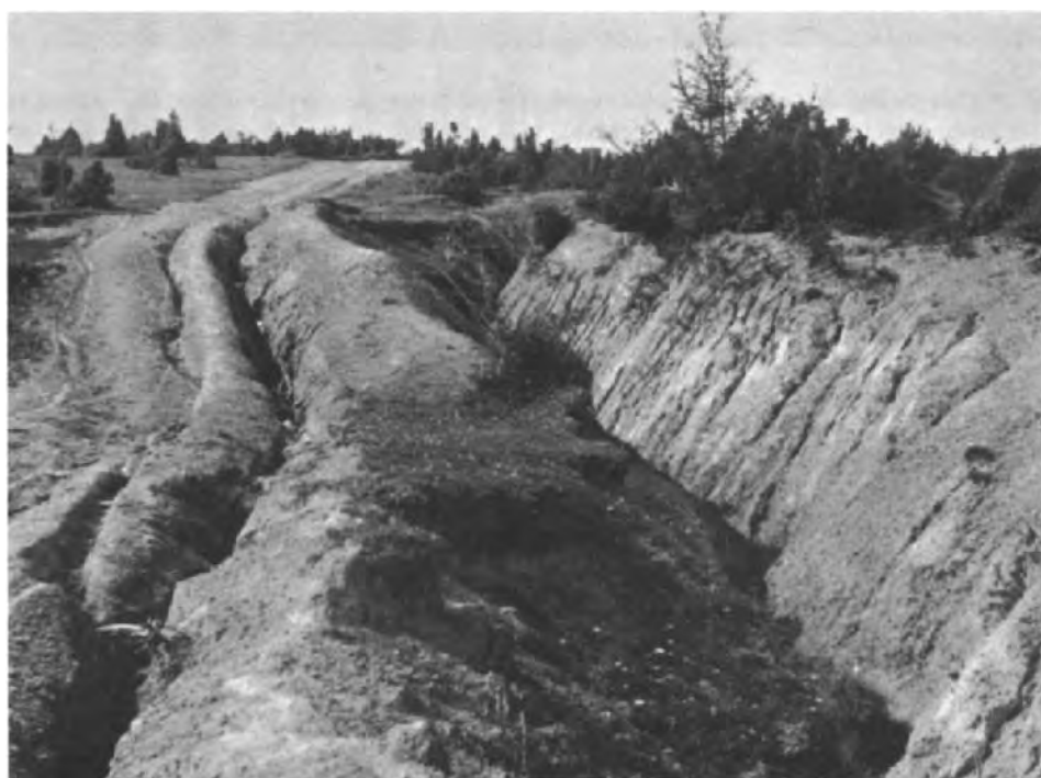
Fig. 18. Road erosion caused by the gouging of tracks and wash (surroundings of Banská Bystrica, Czechoslovakia). (Photo D. Zachar.)
