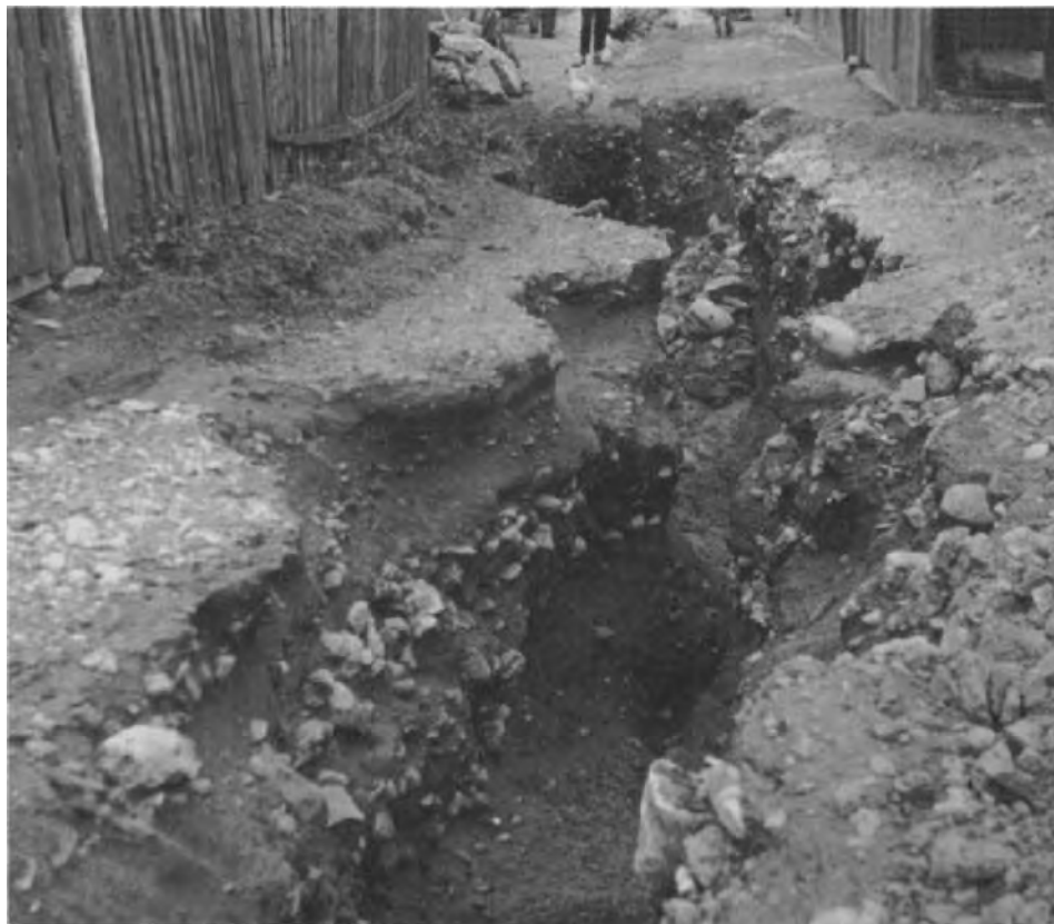
Fig. 98. Road washed by a downpour in the Lučatín community (Czechoslovakia). The gully was 2 m deep in some places. (Photo D. Zachar.)
