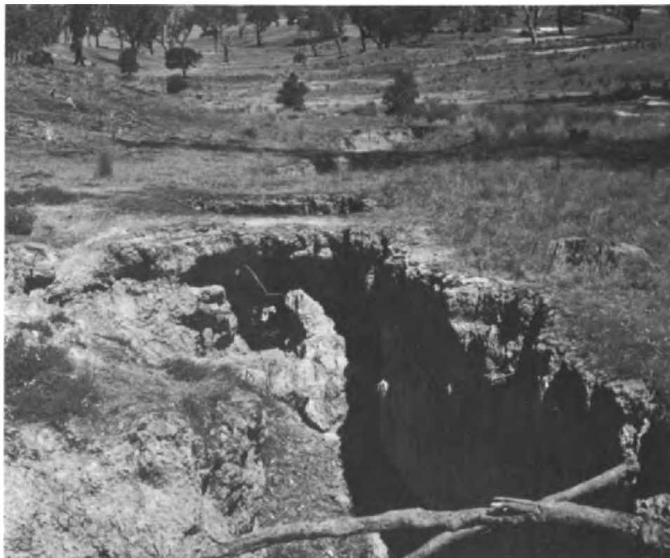
Fig. 36. Tunnel erosion in Ordovician sediments in the central region of Victoria. The funnels, which are connected by an underground corridor, increase in size and after the ceiling collapses they develop into gullies (see also Fig. 25). (By courtesy of Soil Conservation Authority of Victoria, Australia.)
