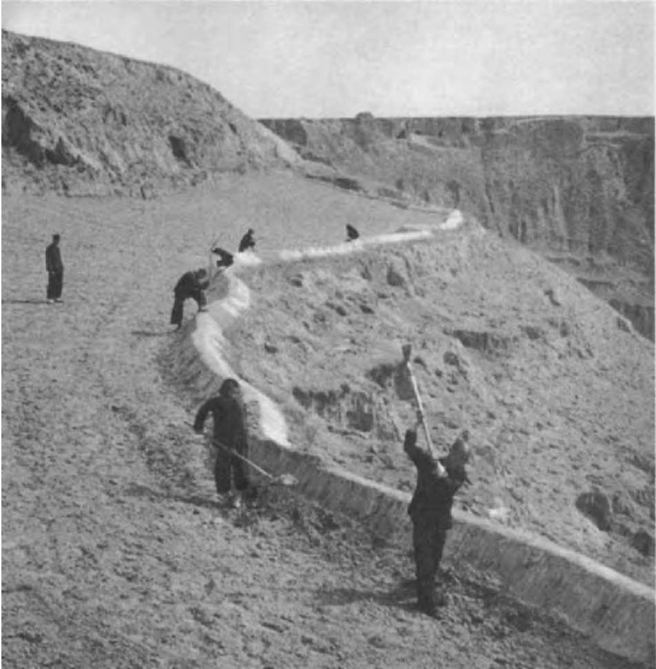
Fig. 162. Erosion control bars for inhibition of erosion on slopes on which agricultural crops are cultivated. (The author's collection of photographs.)
