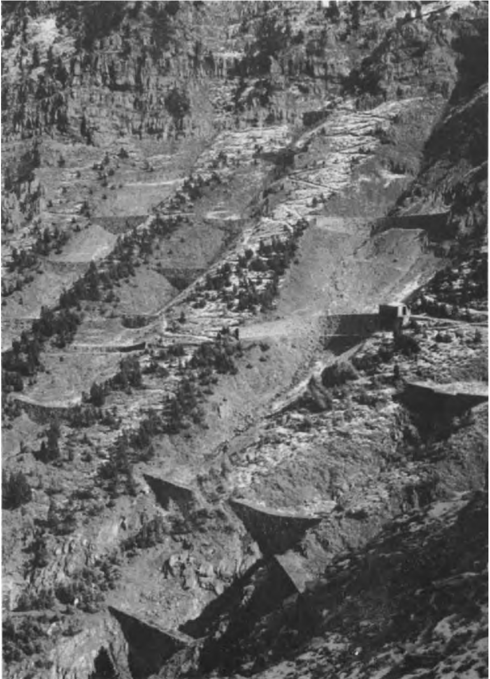
Fig. 156. Protection against rain erosion, snow erosion and avalanches in the Rio Oragon basin, Pyrenees. (Photo F. Rainer.)
