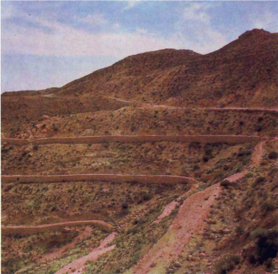
Fig. 174. Antierosive rock terraces in the semiarid region in Tunis. (Photo D. Zachar.)
