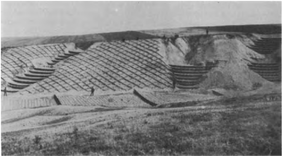
Fig. 144. Soil stabilization by means of a system of technical measures (structures), afforestation, and grass sowing. Neighbourhood of Rakovník (Czechoslovakia). (The author's collection of photographs.)
