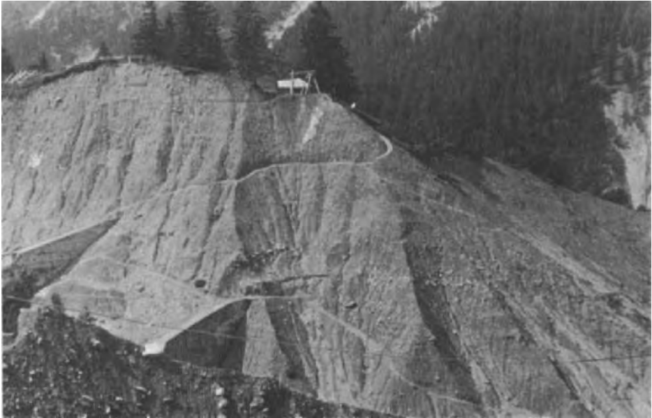
Fig. 154. Stabilization of a ravine bottom together with slope adjustment before surface stabilization (a), soil stabilization by means of willow cordons and grass sowing (b). (The author's collection of photographs.)
