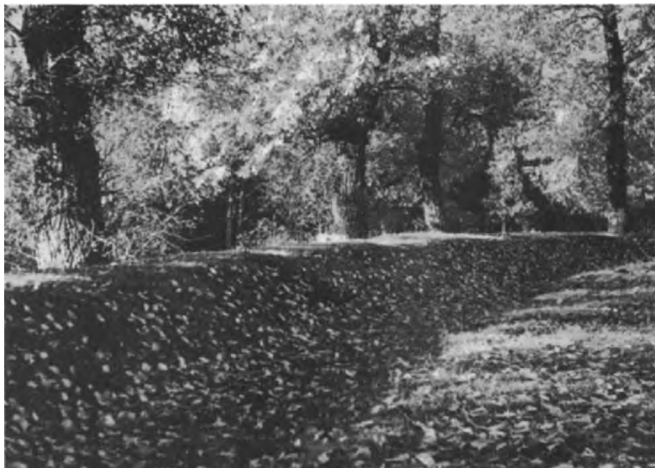
Fig. 141. Erosion control dams built along the banks of ravines (Desna river basin, Ukraine, USSR). (Photo D. Zachar.)
