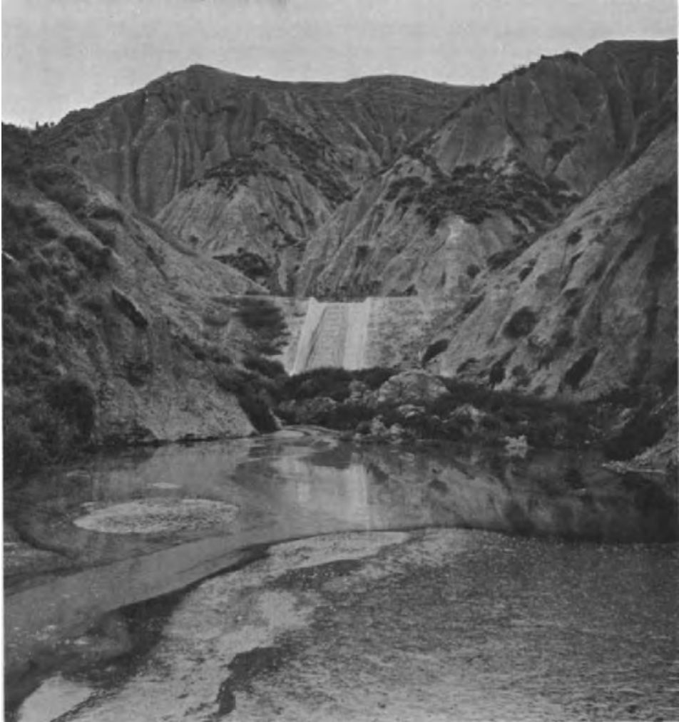
Fig. 150. Flood control achieved by a system of earth dams in the neighbourhood of Pisticci (Italy). (By courtesy of Ente Riforma, Bari.)
