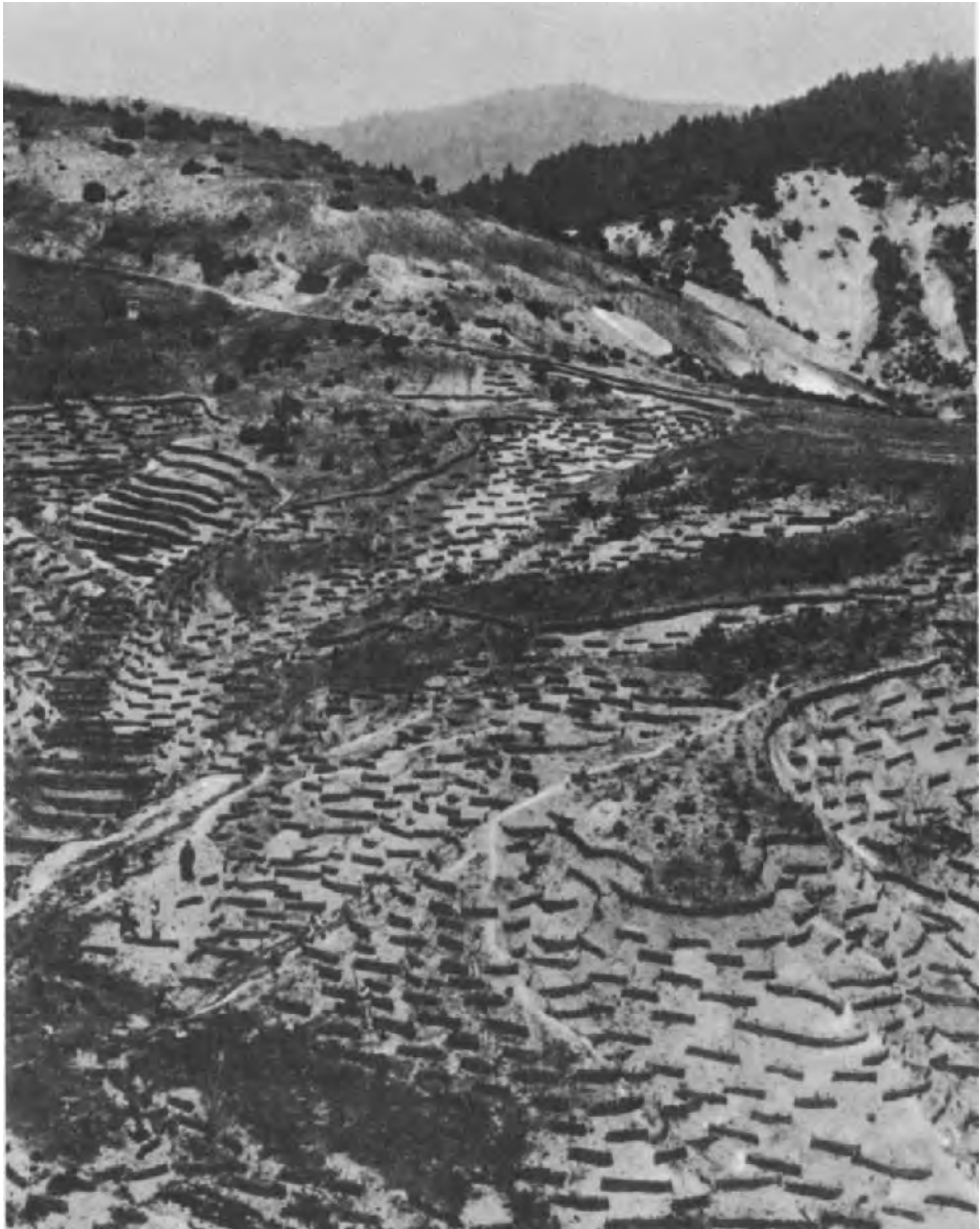
Fig. 146. Stabilization of wasteland by means of fences erected towards the end of the last century. Neighbourhood of Banská Bystrica (Czechoslovakia). (The author's collection of photographs.)
