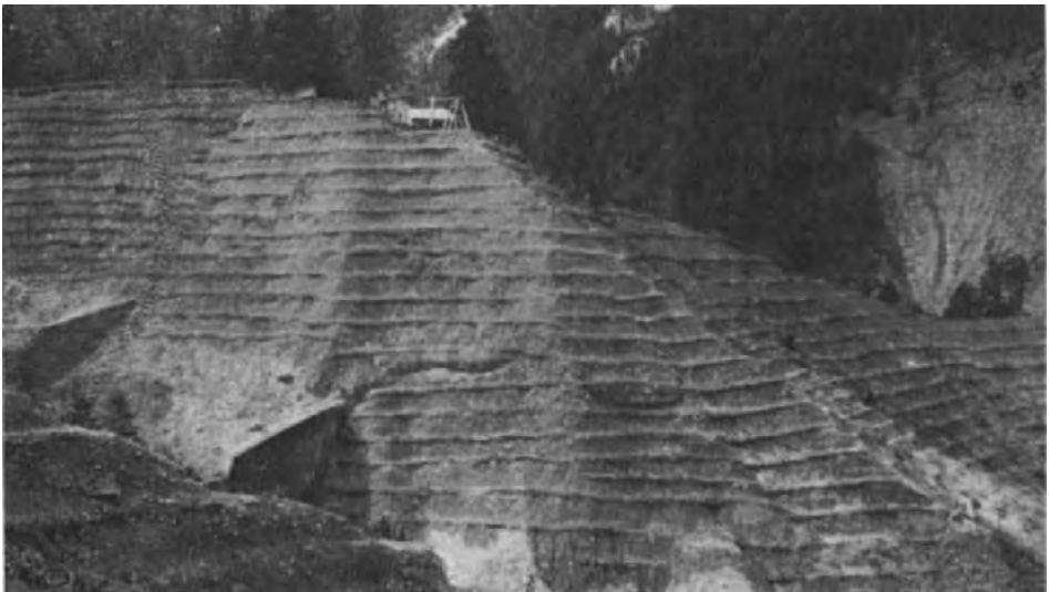
Fig. 154. Stabilization of a ravine bottom together with slope adjustment before surface stabilization (a), soil stabilization by means of willow cordons and grass sowing (b). (The author's collection of photographs.)
