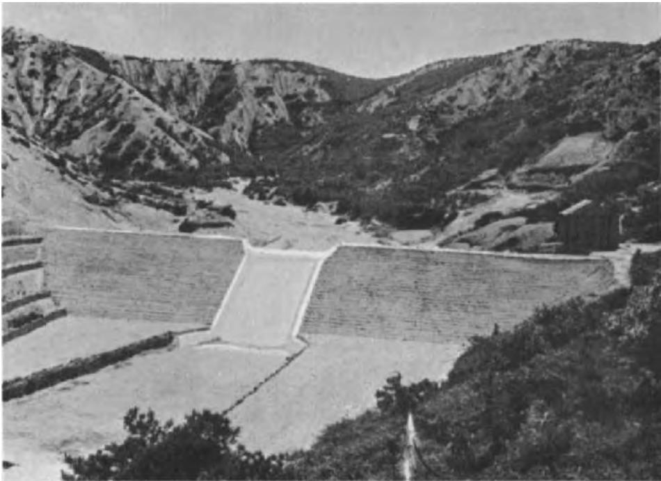
Fig. 165. System of erosion control measures on land destroyed by water erosion, including an earth dam, fences, grass sowing and tree planting (from Conservation in Japan , 1968).
