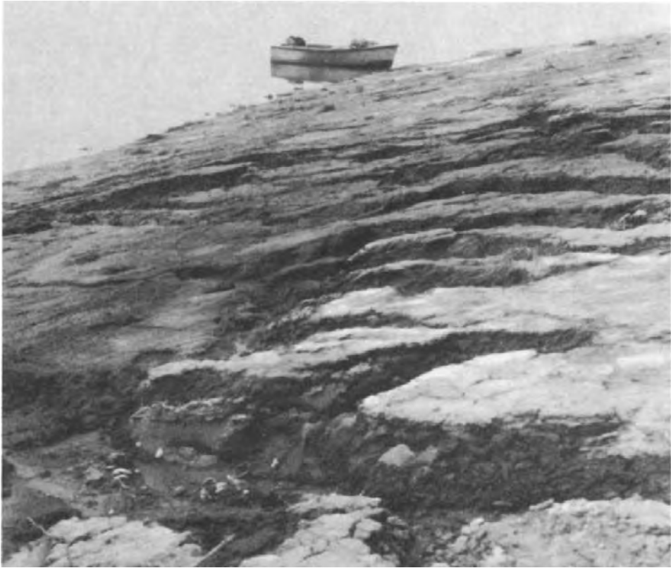
Fig. 10. Soil damaged by lacustrine erosion on the Orava Dam (Czechoslovakia). (Photo D. Zachar.)
