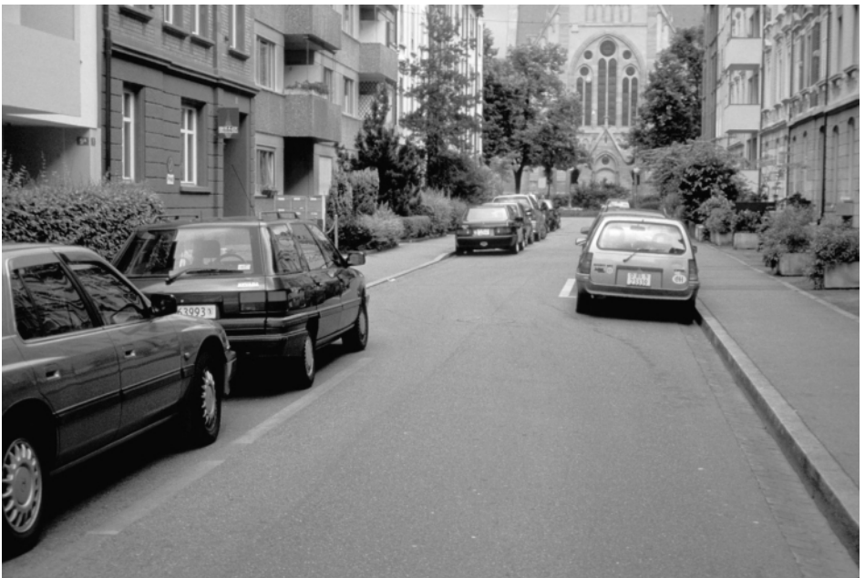
Figure 12.18 Traffic-calming devices: chicanes. Chicanes, as here on a street in Basel, alternate parking and landscaping from one side of a street to the other to slow traffic.
