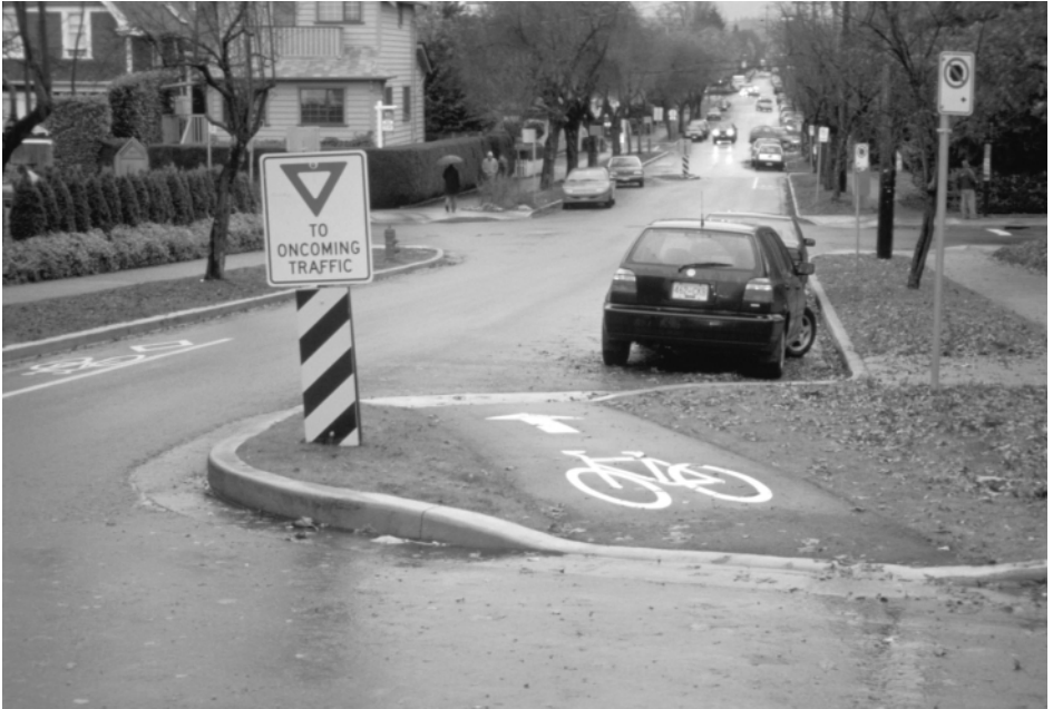
Figure 12.19 Traffic-calming devices: bulbouts. Bulbouts, as here in Vancouver, push out the curb at an intersection to slow traffic.
