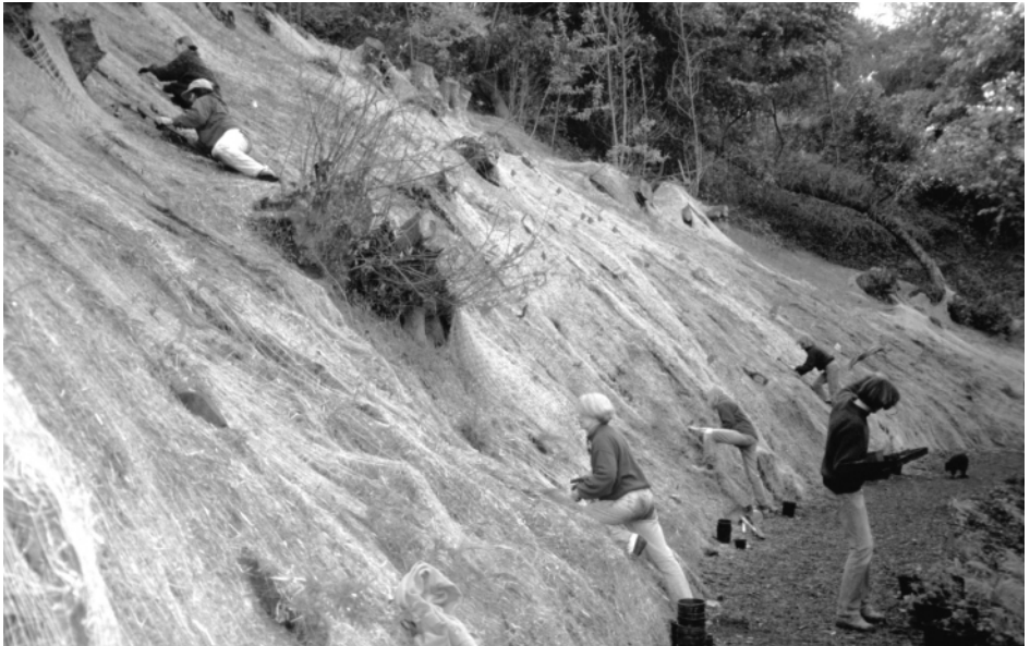
Figure 12.23 Creek restoration. Volunteers plant seedlings of native shrubs along a re-created stream channel for Sausal Creek in Oakland.
