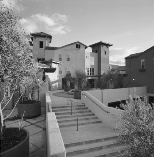
Figure 5.3 Well designed affordable housing. Affordable housing, such as this development in San Jose, can be made attractive and human-scale.
