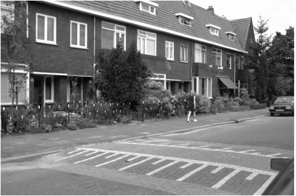
Figure 12.17 Traffic-calming devices: a speed table. Speed tables, as here on a residential street in Utrecht, create a broad, raised area of paving.
