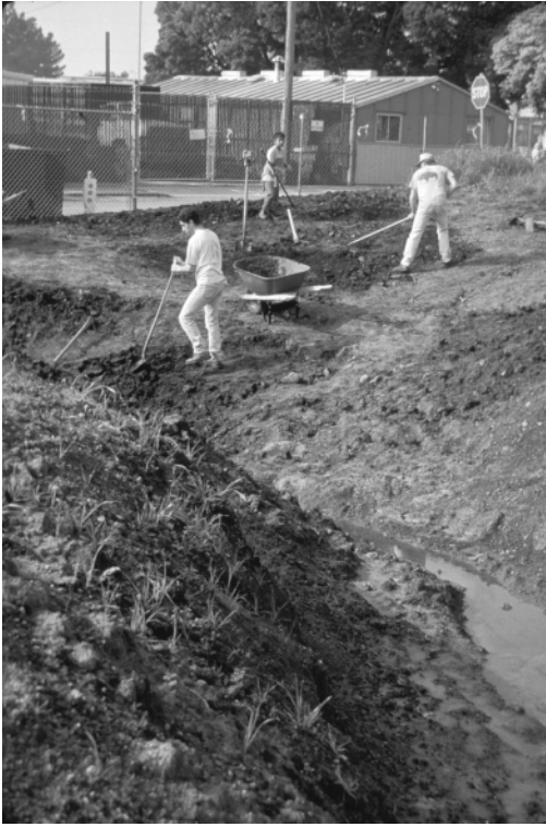
Figure 5.11 A restored stream. Sustainable design instead respects and works with the natural landscape, in this case by unearthing a culverted creek in Berkeley and restoring a naturalistic, meandering stream channel.
