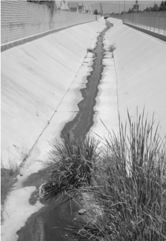
Figure 5.10 A channelized stream. The engineering approach to development has resulted in destruction of natural landscape elements, as illustrated by this channelized stream in Las Vegas.
