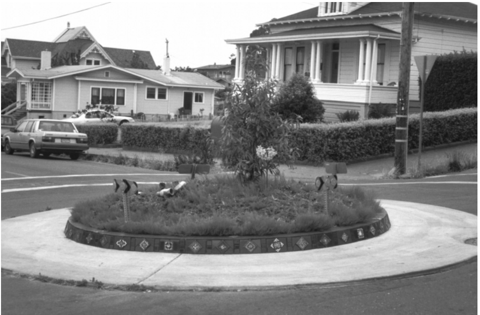
Figure 12.20 Traffic-calming devices: circles. Traffic circles, as here in Arcata, California, force traffic to move more slowly at intersections.
