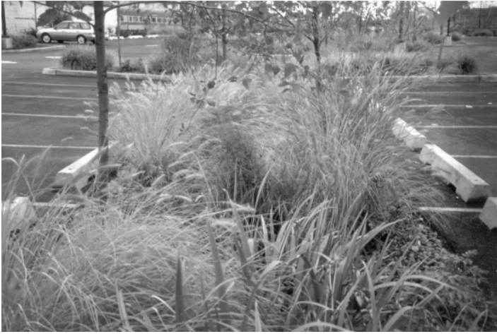
Figure 13.2 Natural drainage swales. Plantings in this parking lot in Portland, Oregon help filter runoff and allow it to drain into the soil.
