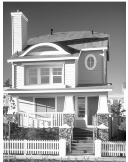
Figure 5.4 Compactly designed single-family housing. Single-family detached housing is possible within compact neighborhoods such as this one in Mountain View, California.
