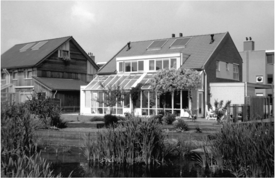
Figure 5.13 Ecological homes. Commissioned by the Dutch Environment Agency, the community of Colonia uses passive solar architecture in many of its 101 homes, as well as solar hot water heating and thick, heat-retaining walls. These and other strategies reduce gas consumption by 40 percent and water consumption by 20 percent.
