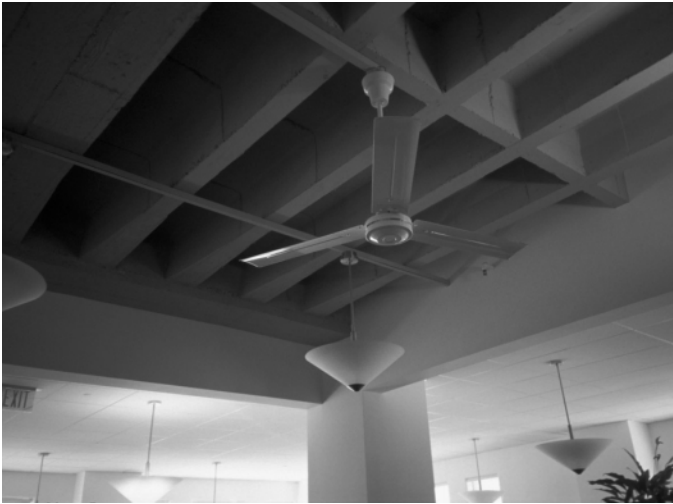
Figure 13.4 Green building strategies can be simple. Ceiling fans promote natural ventilation in Berkeley’s renovated Civic Center building, while high ceilings and large windows let in daylight, reducing artificial lighting needs.
