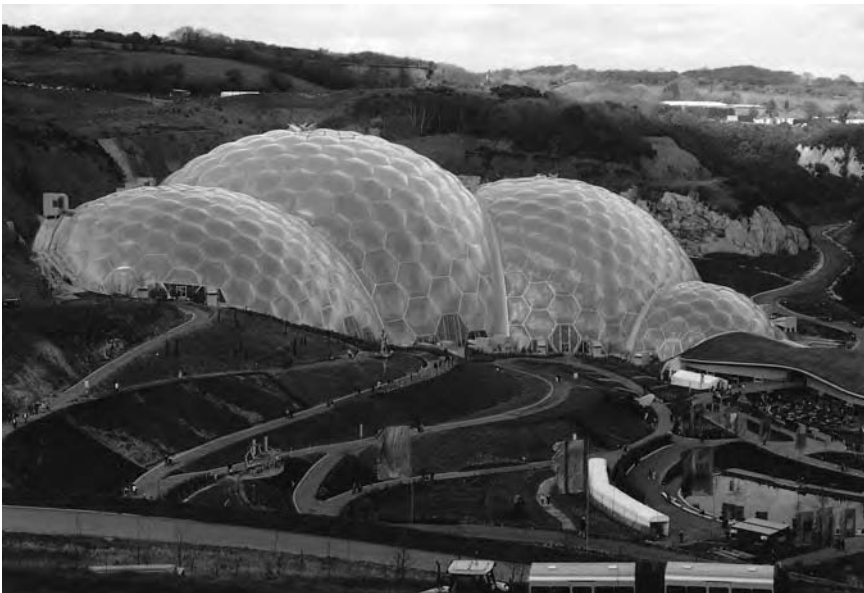
Fig. 3.5 The giant biomes of the Eden Project in the former Bodelva pit.
