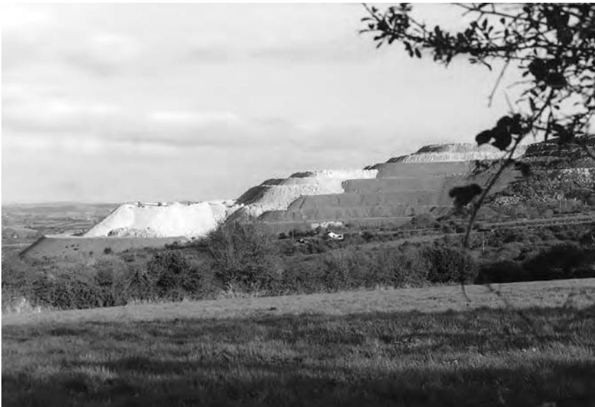
Fig. 3.3 The distinctive visual and environmental impact of a multi-lift benched waste tip from Goonbarrow China Clay Works.
