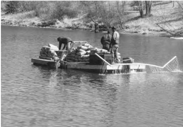
Alum in powdered form is often used for pond projects. It can be mixed with lake water and added as a liquid slurry through a PVC pipe manifold. A light dose would be 100 pounds of alum per pond-acre. Often, a higher dose is used.
