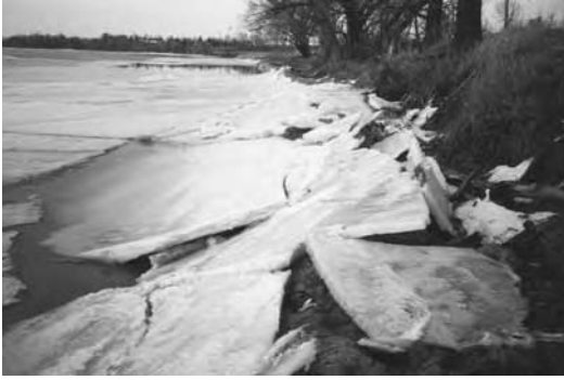
Although damage from ice action is usually minor, it can be severe in some winters. (From Minnesota Department of Natural Resources.)
