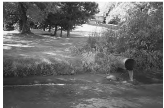
A significant difference between natural ponds and constructed ponds is the type of water that feeds into them. Stormwater treatment ponds often receive higher nutrient loads than natural ponds.
