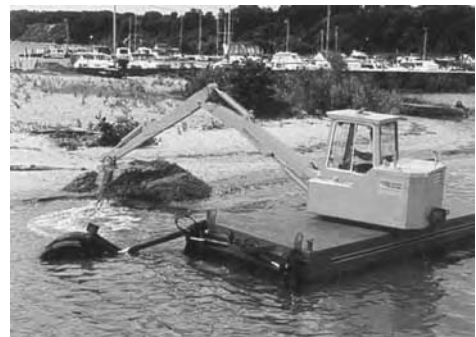
The pontoon wheels help stabilize the excavator in the water.
