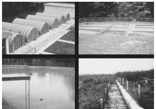
A number of options are available for centralized treatment, including fixed film processes (upper left), aerated lagoons (upper right), facultative lagoon (lower left), and wetland treatment (lower right). (From USEPA, 1980a.)
