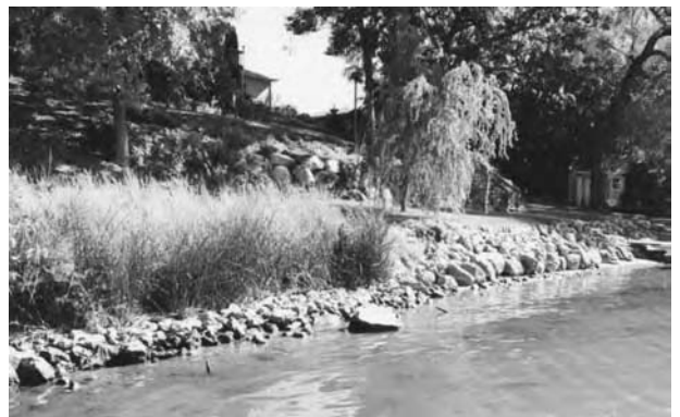
You can use the charts in this section to determine the right size rock for toe protection and then use biostabilization techniques above the waterline. The vegetation associated with biostabilization offers better buffering and wildlife habitat than a fully riprapped lakeshore.
