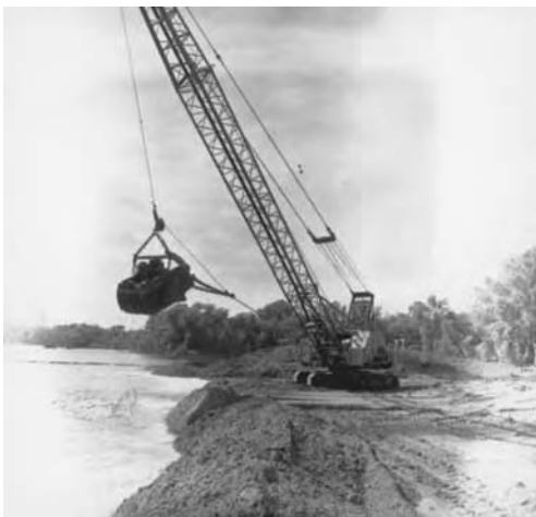
An example of a large-scale mechanical removal technique is this dragline operation. Small-scale mechanical removal techniques rely on the same basic principle: scoop out the muck.
