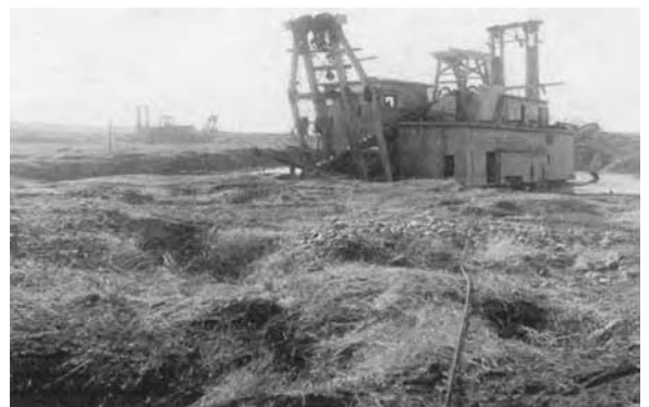
Hydraulic dredge used for placer gold mining in Colorado around 1900. (From Western History, Denver Public Library, Denver, CO. With permission.)
