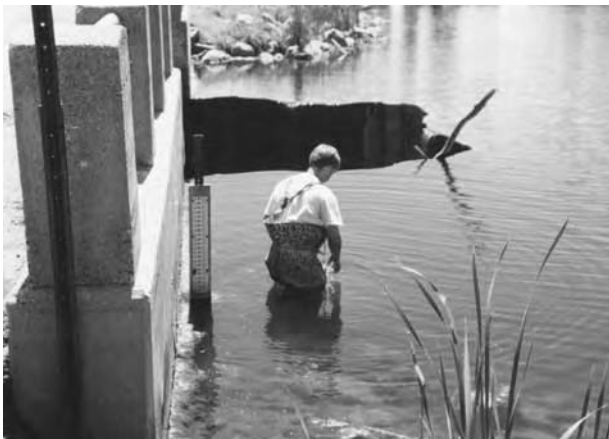
A siphon system is generally cheaper than pumping, but also slower. This worker is checking a site to see if a siphon system will work. Tubes could be placed in the lake and hung over the semi-circular dam. There is about a 10-foot drop over the dam and the lake could be lowered about 7 to 9 feet.
