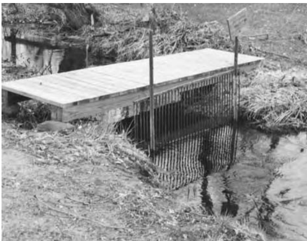
Fish barriers are used to shut off carp runs into shallow spawning areas connected to a lake.
