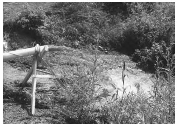
In an ideal setting, you might have a natural depression in an upland area that is not a wetland, close to your dredge site... like the location shown here. Good luck! These settings are rare.
