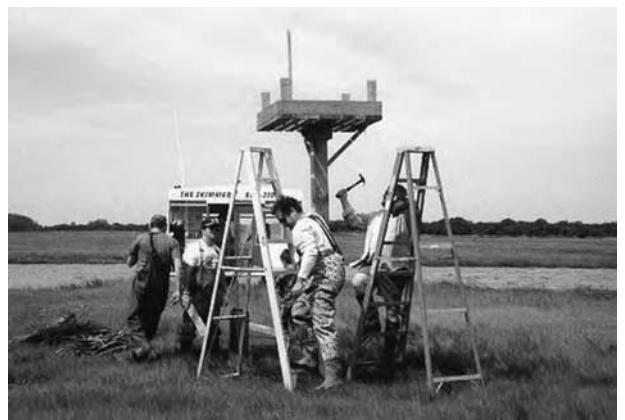
Volunteers erecting an osprey platform in a salt marsh in New Jersey. In the salt marsh, platforms only need to be about 8 feet high. (From Linda Carlough.)
