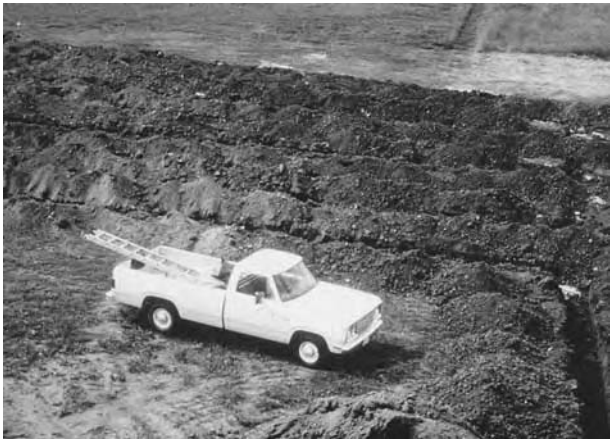
Community drainfields for cluster systems can become quite large. Careful design and construction are necessary to avoid groundwater contamination. (From USEPA, 1980a.)
