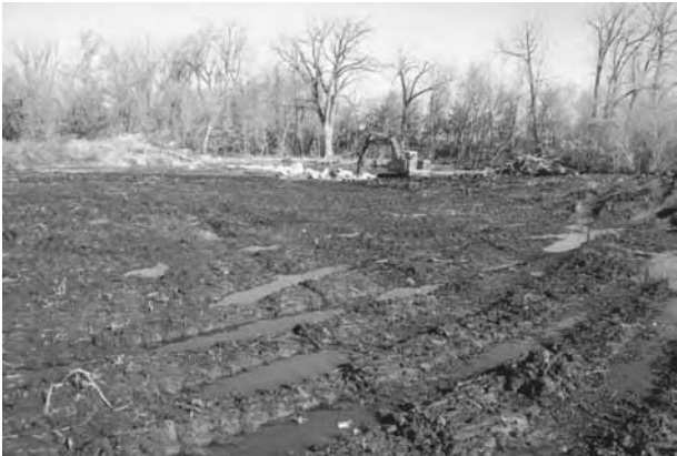
Working in a lakebed without the lake is an efficient way to remove lake sediment.
