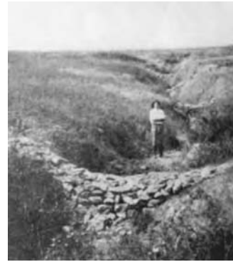
“Series of loose rock dams in a farm gully.” (From Ayres, Q.C., Soil and Erosion Control , McGraw-Hill, New York, 1936.)
