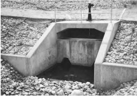
The easiest way to draw down a lake is if it already has some type of flow release system. This lake in Illinois has a bottom release system that can readily lower the lake.
