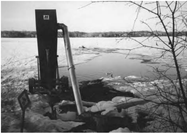
Lake water goes in at the top of the baffle and cascades back into the lake. (From City of Lakeville, Minnesota.)
