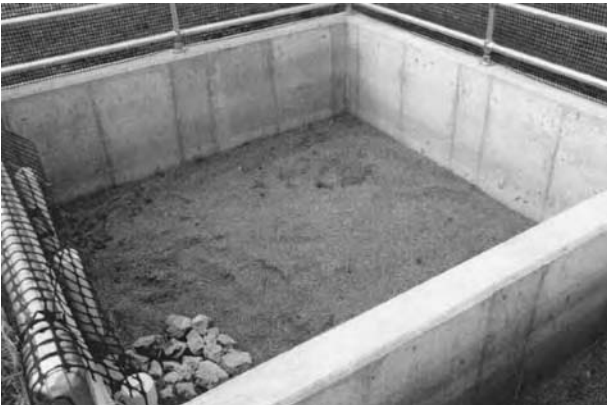
Sand filter ready to filter water from a wastewater pond. Sand filters are sized based on flow. (From Thatcher Engineering, Minneapolis, MN.)
