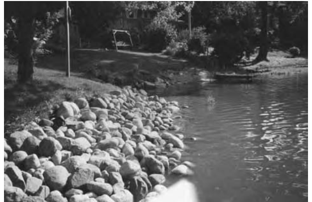
Conventional riprap revetment uses rock to dissipate the wave runoff energy. In many cases, riprap can be converted to rootrap. Thin out some rock above the waterline and add 4 to 6 inches of soil. Place an erosion control mat on top of the soil and plant the area with native vegetation.
