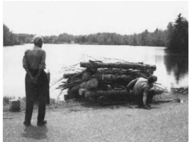
Log cribs are an example of artificial structural habitat. Cribs should be made of green wood (it is less buoyant than dry wood) and weighted down with 300 pounds of clean stone. (From Fish America . With permission.)
