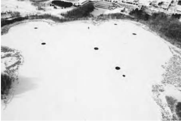
Winter diffuser aeration system operating on a 75-acre lake. An aerial view shows seven diffuser heads spread around the lake with the intent of aerating small pockets in the lake. (From H.B. Huller, Company Nature Reserve, Vadnais Heights, MN.)
