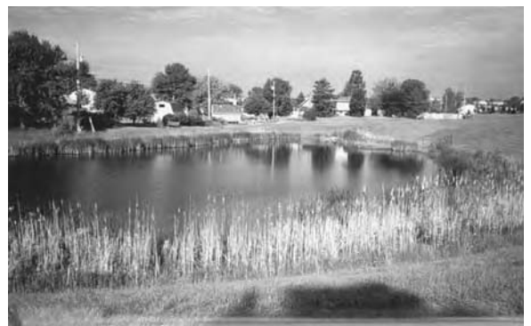
This 20-year-old constructed pond is used as a sedimentation pond to treat stormwater runoff. However, with a combination of watershed and lake projects, it functions like a natural pond.
