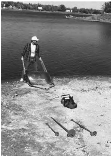
The slusher sediment removal system consists of a slusher, a winch, and land anchors.
