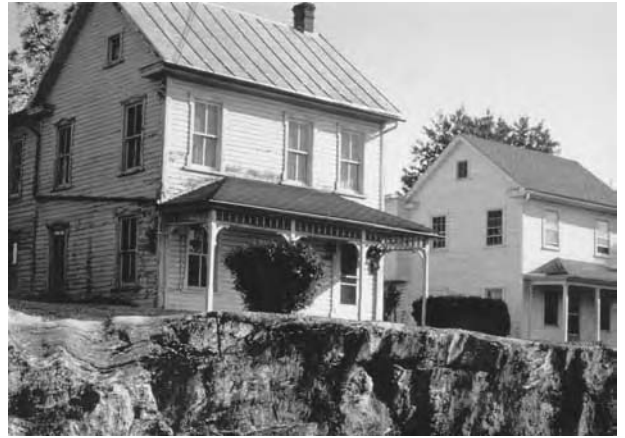
Shallow bedrock poses problems for conventional on-site treatment systems. Sometimes, mound systems will work. (From USEPA.)
