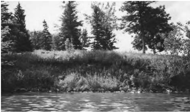
For this high-bank, low-energy setting, erosion was controlled using permanent shoreline wavebreaks in the form of footer stones. The bank is reshaping itself to a stable configuration and vegetation is becoming reestablished on its own.
