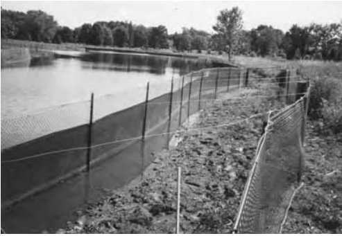
If birds or waterfowl are a serious problem, it takes extra effort to exclude them from new plantings. Here, fencing and wire were used to dissuade grazing of new plantings by birds.
