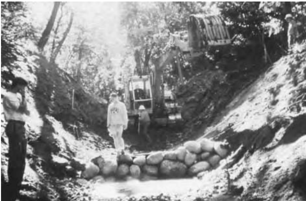
Reducing the gradient in gullies or ravines reduces the erosive force of the water flows. Grade control structures such as this rock weir reduce flow velocities and allow a streambank to reestablish vegetation and stabilize. The rock weir is constructed in the shape of an arc with the high point oriented upstream.
