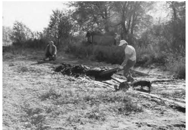
Winch the load to high ground. You have to tip over the slusher to empty the bucket. The next step is to haul away the dredge spoils.
