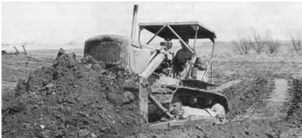
Stormwater ponds are constructed for water-quality purposes, not for fishing. Constructed fishing ponds should be at least 10 to 15 feet deep over one fourth of its area. (From Pond Management in Oklahoma, Oklahoma Department of Wildlife Conservation, 1984.)
