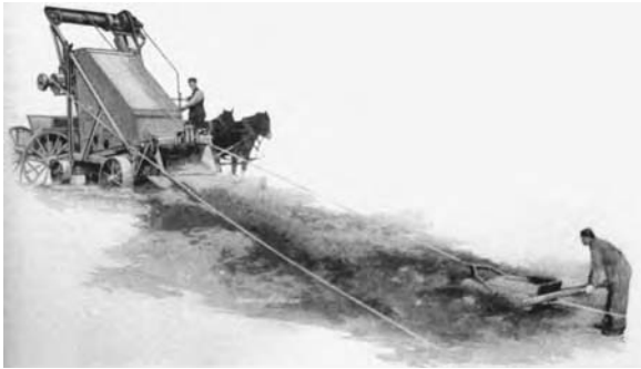
A powered road scraper, referred to as the Albrecht Excavator. (From Excavating Engineer , 12 (March), 207, 1916.)
