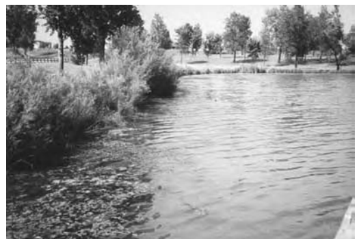
Sometimes, stormwater treatment ponds will exhibit excessive algal growth due to high nutrient loads. Also, because new ponds do not have a native aquatic plant seedbank, invasive plants may dominate and produce nuisance conditions.
