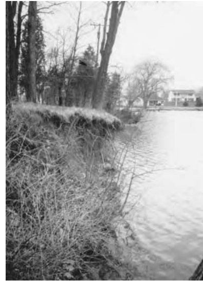
What can be done to stabilize this high-bank, low-energy condition? Probably toe stabilization, followed by bank reshaping.
