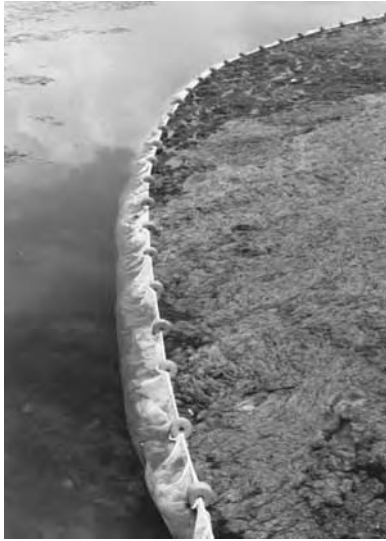
The other end of the net is drawn in. Floats spaced every 18 inches or closer should prevent the algae from overtopping.
