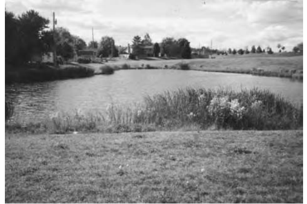
A wet pond in Lakeville, Minnesota, used for stormwater treatment. Sometimes, stormwater ponds can be manipulated to be both a stand-alone water resource and a stormwater treatment system. Additional ideas on storm pond management are found in Chapter 7.
