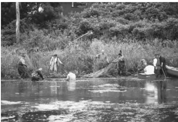
A reinforced fish seine can remove soft sediments in nearshore areas. The lead line (bottom line) bites into the sediments and scrapes off 0.5 to 1.0 inch of sediment per haul. A short net, 5 to 10 feet long, works better than a longer net.
