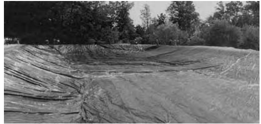
Geomembranes are one option for sealing a leaky pond bottom. The geomembrane should be covered with 6 to 12 inches of sand.
