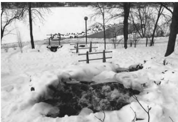
When the pump-and-baffle system is built into a hillside and uses natural rock for baffles, it mimics a bubbling brook. It looks natural and is a permanent setup, but can cost $30,000 or more.
