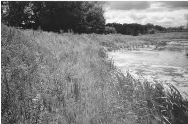
This 5-year-old constructed pond attracts a variety of wildlife and serves as a water-quality treatment pond. The shoreline and shallow-water areas were planted with native plants.
