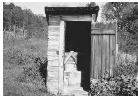
The old outhouse has a role in some settings. If the pit is lined and it can be pumped, it is an on-site option. (From USEPA.)
