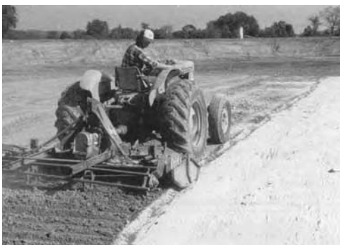
Bentonite, a swelling clay, is mixed with soil and then compacted. This forms a bottom seal for a pond. (From Tourbier, J.T. and Westmacott, R., Lakes and Ponds, 2nd ed., ULI, The Urban Land Institute, Washington, D.C., 1992. With permission.)
