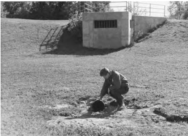
Outlet pipe of dry pond with emergency outlet in the background.
