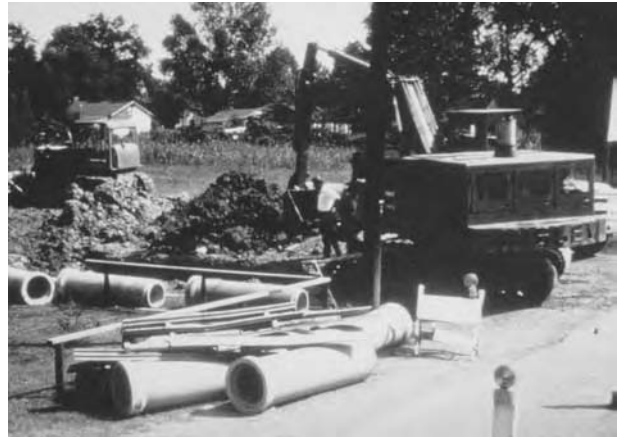
In hilly terrain, deep cuts may be necessary to make gravity sewers flow; otherwise, expensive lift stations are needed. (From USEPA, 1980a.)
