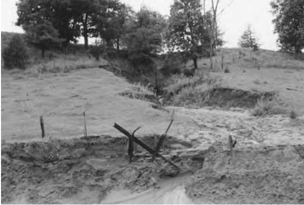
Gully erosion is another form of streambank erosion. The keys to stabilization are to stop head cutting, reduce the gradient, and revegetate.
