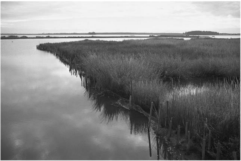
Fig. 9.3 Restoration of saltmarsh by sediment deposition. The area on the right was open water a year before the photograph was taken, the original saltmarsh having been lost due to erosion initiated by introduced nutria/coypu. The saltmarsh has been restored by pumping sediment into areas cordoning off using wooden stakes with haybales tied to them and planting this with smooth cordgrass, Spartina alterniflora (Blackwater National Wildlife Refuge, Maryland, USA).
