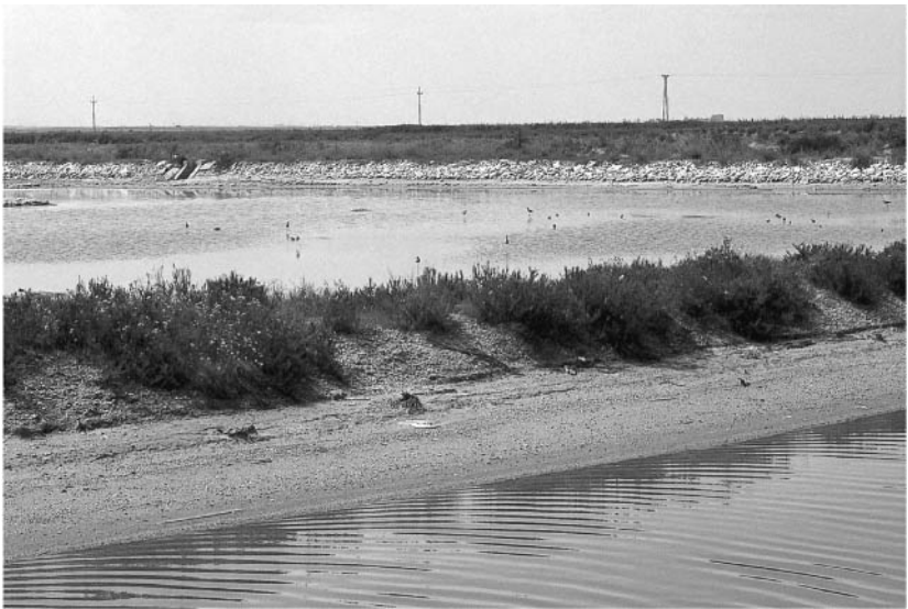
Fig. 9.9 Salinas/salt evaporation ponds/solar ponds. These are artificial, shallow, saline lagoons used for salt production in hot climates. Seawater is passed through a series of lagoons, during which process it becomes increasingly saline due to evaporation. Eventually the salt crystallizes out on the final set of lagoons and is collected. Salinas support a similar assemblage of specialized birds and invertebrates to those found in natural, high-salinity lagoons (Margherita di Savoia, Puglia, Italy).
