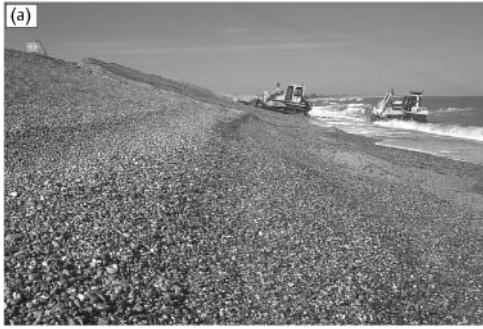
Fig. 4.10 Sea-level rise and freshwater and brackish habitats. This shingle bank was artificially maintained to protect the important saline lagoons and freshwater reedbed behind it (a), but breached 2 years later ((b) was taken from a similar position).
