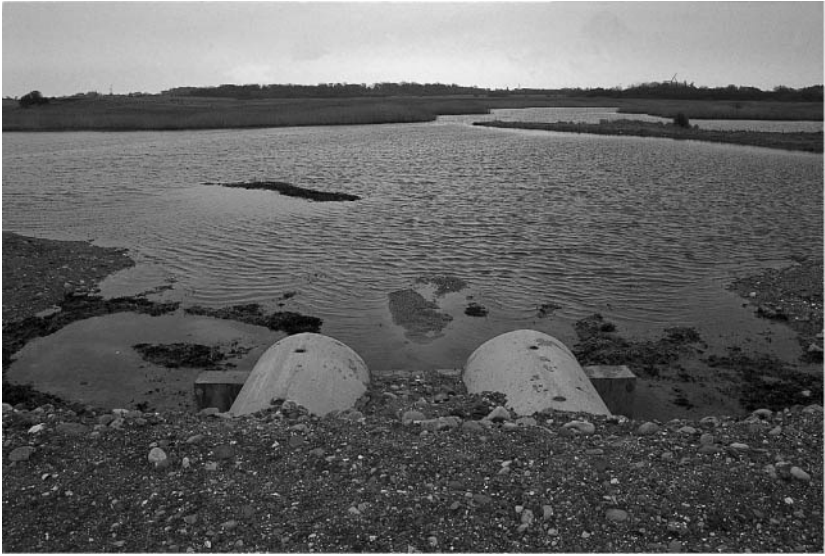
Fig. 9.11 Reducing nutrient levels in saline lagoons. Nutrients levels in this lagoon are high due to large inputs of agricultural run-off in the freshwater that drains into it. Two projects are being used to address this. The first involved increasing exchange of water through a shingle bank that separates the lagoon from the sea, to help flush out nutrients that have accumulated in the lagoon. The second involved creation of a 54-ha shallow freshwater lake and 14 ha of grassland on former agricultural land within the catchment. This aims to reduce the area of arable from which nutrient-rich run-off can occur and to retain nutrients within the run-off before they reach the saline lagoon (Tryggelev Nor, Fyn County, Denmark).
