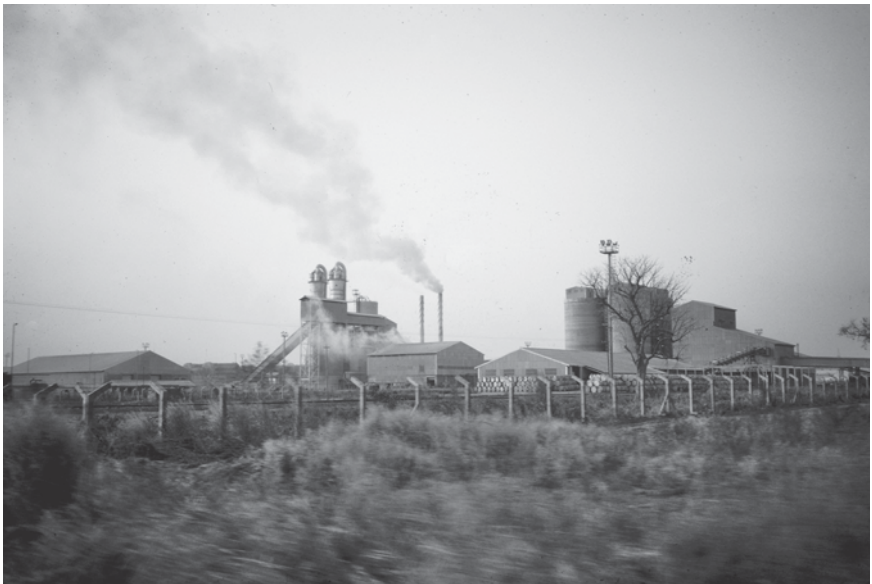
Plate 12.3 Cement factory, Nigeria. Cement is critical to building projects in the developing world, and often has to be imported. Yet, like so many other products, its manufacture can bring significant environmental problems, generating large amounts of CO 2 as well as particulate matter, nitrogen and sulphur oxides, volatile organic compounds and heavy metals.
