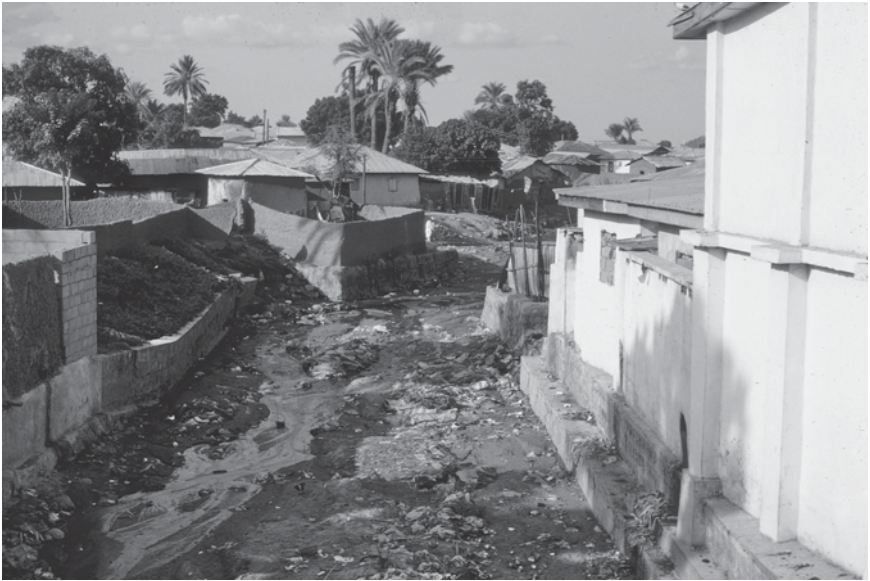
Plate 12.1 Rubbish-blocked urban stream channel, Nigeria. Problems of municipal waste disposal, poor-quality water supplies and flooding are connected and form a major challenge to raising living standards in developing-world cities.
