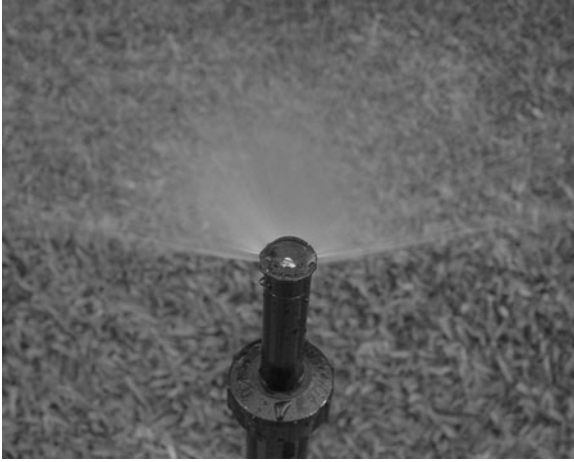
Fig. 7.9. Fixed sprinkler heads usually operate at low water pressure, producing a fine spray covering a small area.
