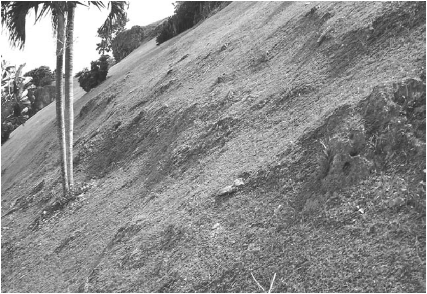
Fig. 1.2. Established turf on the steep slope effectively prevents soil erosion.
