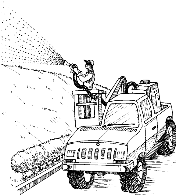
Fig. 4.8. In hydroseeding, seeds, paper pulp and fertilizer mixed with water are sprayed onto the soil surface from a distance.
