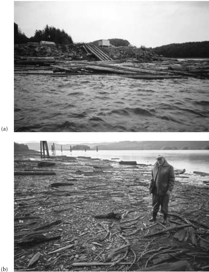
Fig. 15.1 (a) Ramps used to slide logs from trucks into an estuary on Skidegate Channel, Queen Charlotte Islands, BC, Canada. (b) Accumulation of wood fragments and debris at the base of a log dump ramp used for several decades at Bearskin Bay, Queen Charlotte Islands, BC, Canada. (Photographs taken in August 2000, courtesy of Ray Sjolund, Department of Fisheries and Oceans.)
