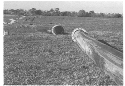
Figure 8.7 Flanges welded to pipes in the field ready for final positioning and bolting together (Courtesy: Vinidex Tubemakers P/L)
