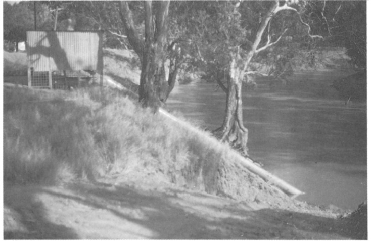
Figure 8.13 This structure takes water under a natural floodway
