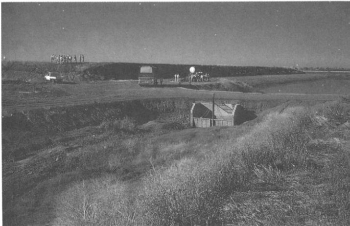
Figure 5.8 Tailwater is collected in a sump, and pumped into the adjacent storage dam.
