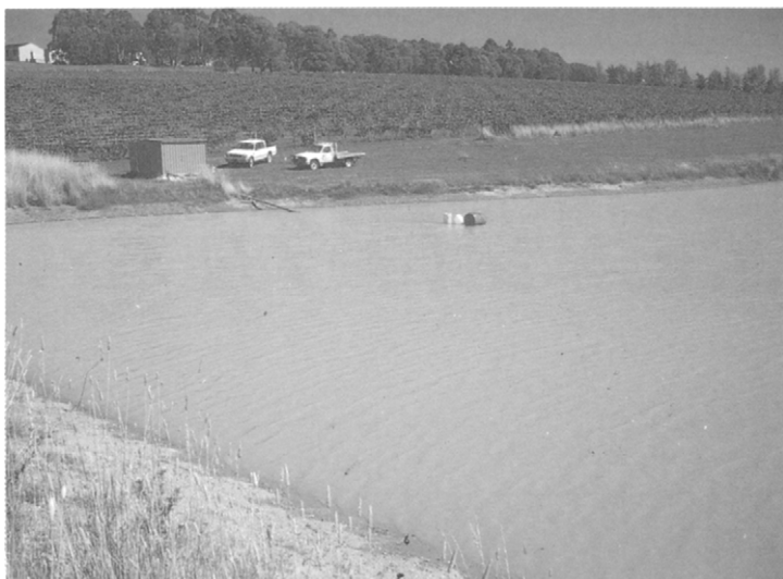
Figure 8.1 On this vineyard, the water supply and pump station are conveniently adjacent to the irrigated area, minimising costs of water reticulation. Water is delivered first to the top of the hill, then submains bring the water downhill to the laterals, to ensure even pressure to the laterals.
