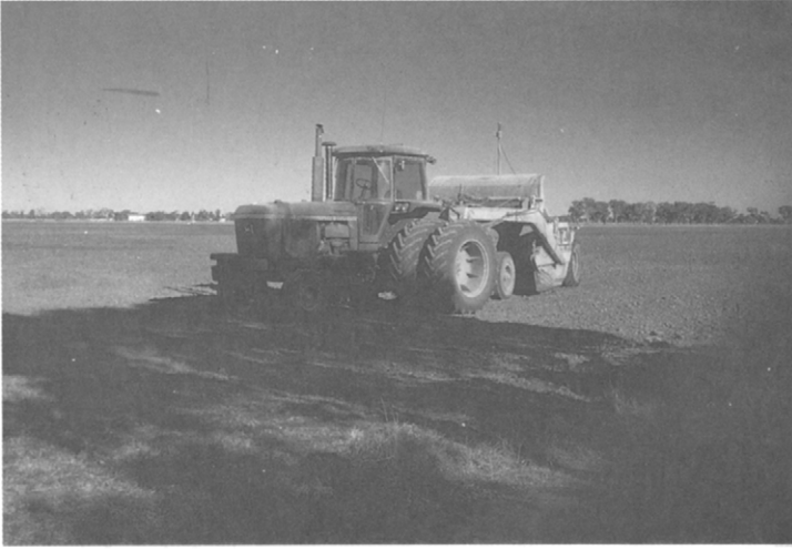
Figure 5.5 Earthmoving under way using a tractor drawn scraper. The operating height of this is adjusted in response to a laser signal. The mast on the machine carries the laser receiver; the laser emitter is mounted on a tower near the centre of the field.
