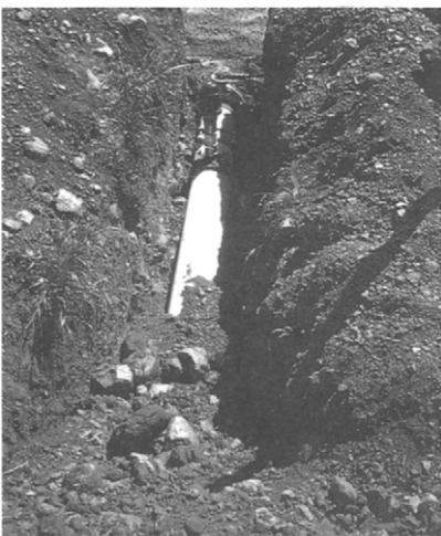
Figure 8.10 Concrete thrust blocking prior to completion of backfilling
