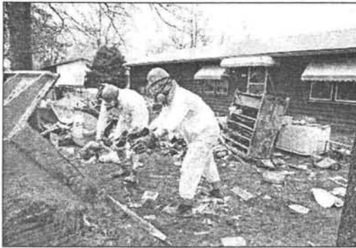
Fig.3. Two Workers Wearing Gas Masks and Protective Clothing Loading Debris Contaminated by Dioxin into Tractor Trailers
