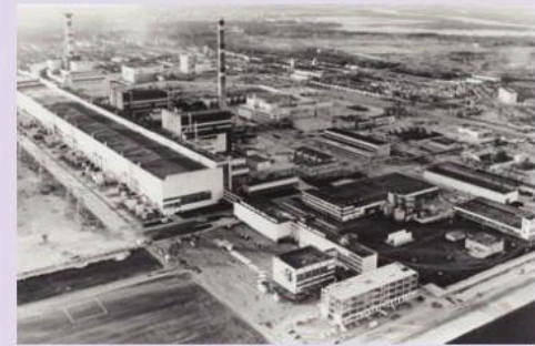
↑ When this nuclear power plant exploded it scattered radioactive uranium across the surrounding countryside.
