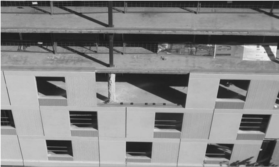
FIGURE 9–2–9 Precast panel installation process.
