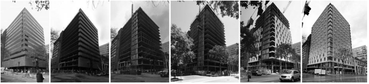
FIGURE 9-2-3 Sequence of building process. (See color insert for full color figure.)
