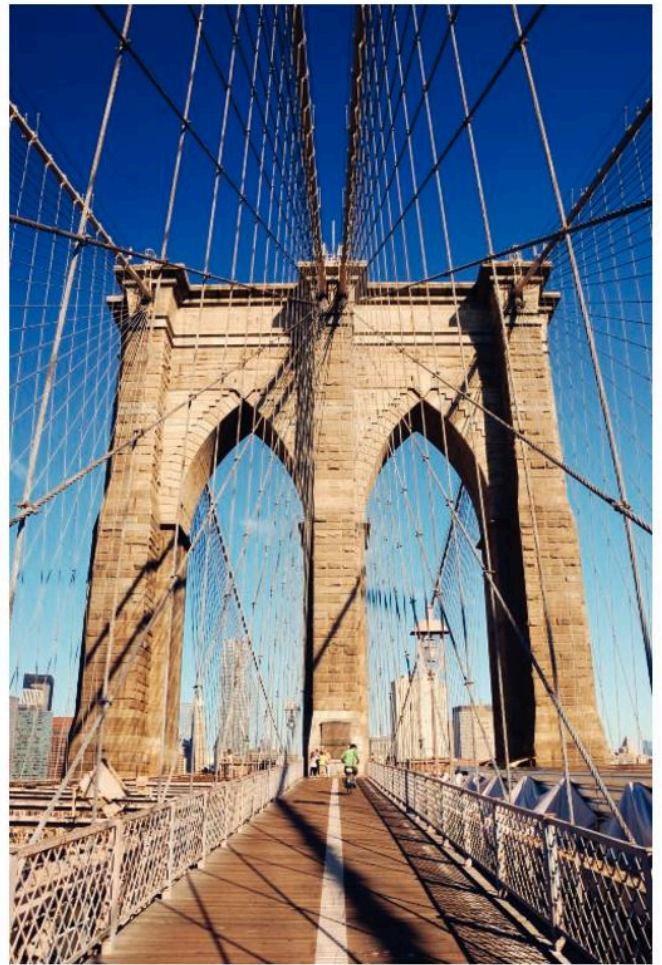
Brooklyn Bridge in America
