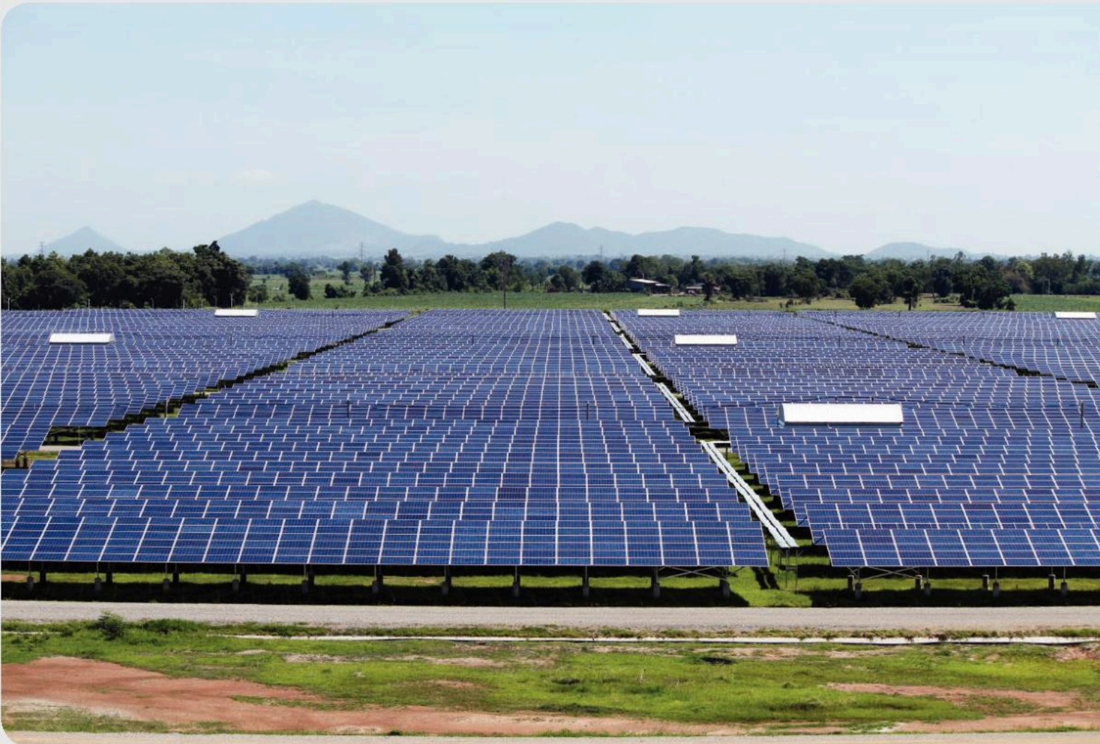
▲ A solar farm
