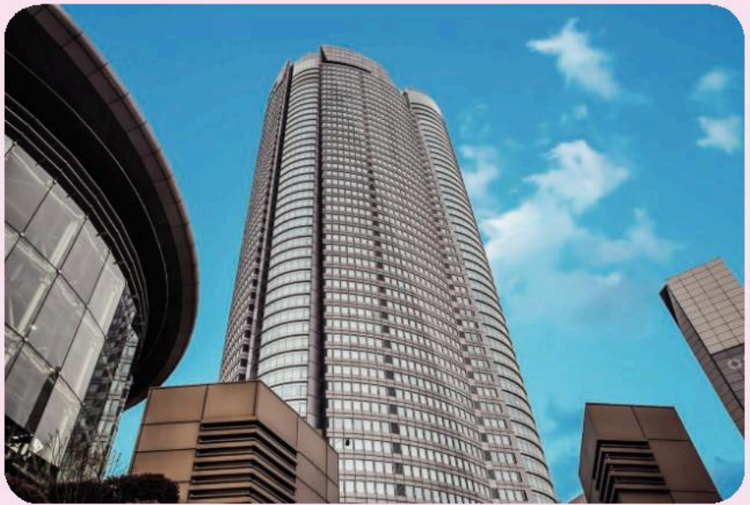
▲ The Roppongi Hills Mori Tower is one of Tokyo's tallest buildings. The foundations are built with oil-filled shock absorbers that control the swaying of the building in an earthquake
