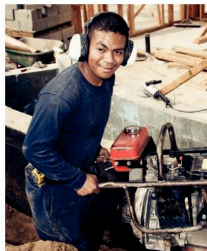
These ear defenders will protect the worker from the damaging sound energy emitted from the equipment he is operating
