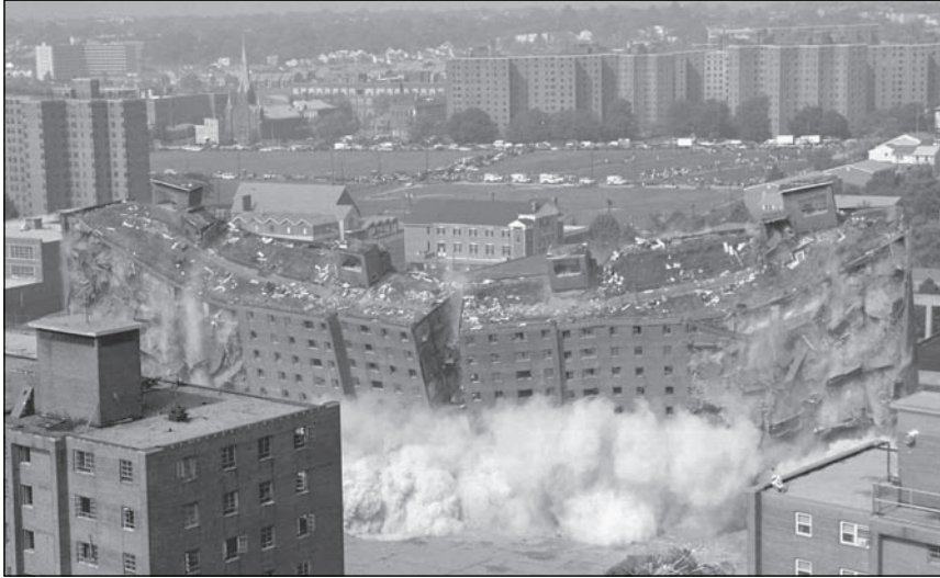
Since the dynamiting of Pruitt-Igoe in 1972, a similar fate befell other high-rise public housing as city governments attempted to correct past mistakes (not considering social as well as physical factors) with low-rise replacements. This photo shows the implosion of one of three remaining 13-story buildings of the Scudder Homes complex in Newark, New Jersey, in 1996.
