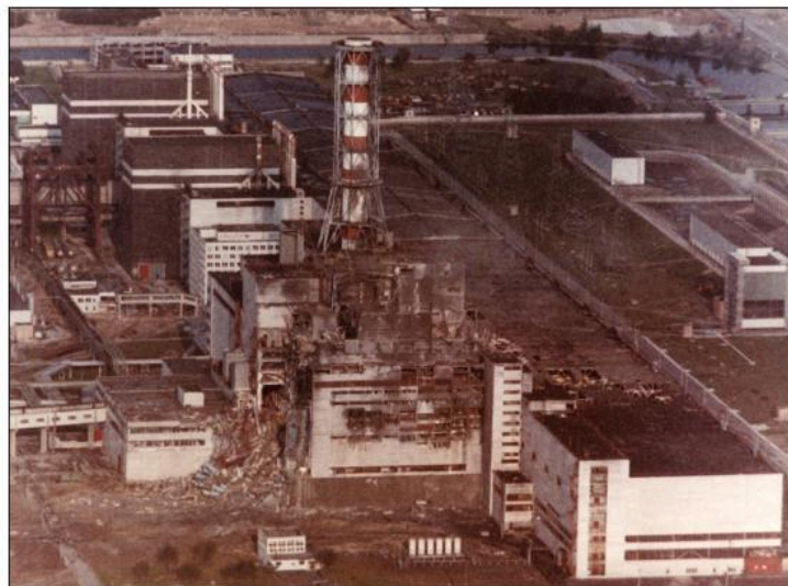
▲ Figure 1.1.2 The Chernobyl nuclear reactor plant after the explosion in 1986
