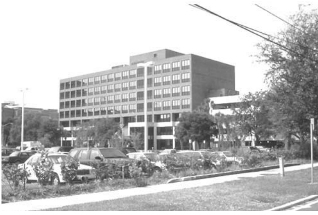
Figure 28.6 Vegetation blocks views to this health facility's main parking structure and its entrance.
