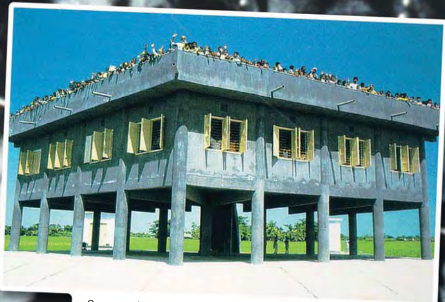
Concrete shelters constructed on stilts, as shown here, and reinforced school buildings are refuges from high floodwaters and winds that can knock down all but the strongest buildings.
