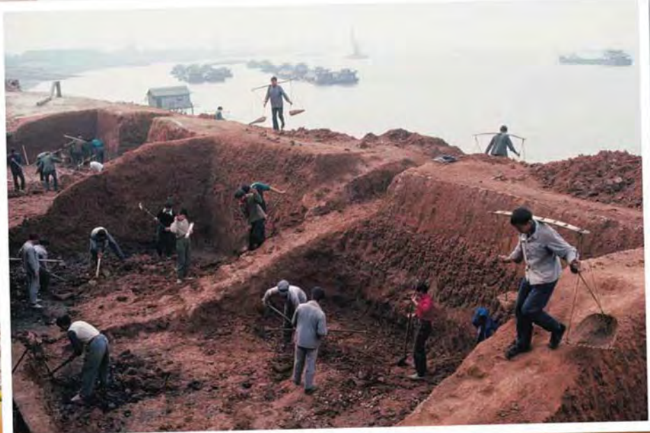
Along the Chang Jiang, human labor is still essential for flood control. These laborers work with shovels and other tools to fortify the banks of the river with dirt to prevent flooding.
