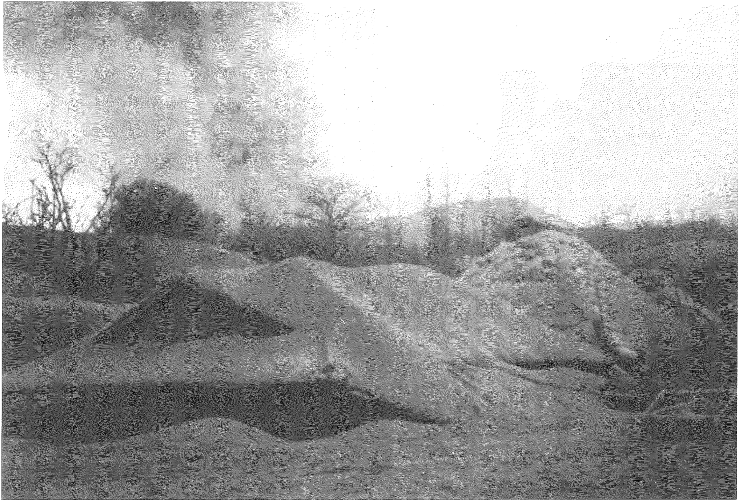
Fig 5.6. Buildings partially buried by volcanic ash during the 1914 eruption of Sakurajima, Japan.
