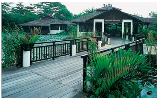
A boardwalk at Sungei Buloh Wetland Reserve
