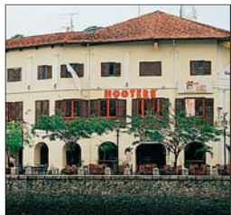
Clarke Quay's refurbished warehouses
