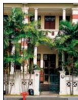
The Art Deco Style (1930–1960) shophouse is typified by Classical geometric motifs, as seen in this unit (No. 30) on Bukit Pasoh Road.
