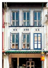
The First Transitional Style (early 1900s) shophouse is three storeys high, as shown by this unit at Telok Ayer Street.
