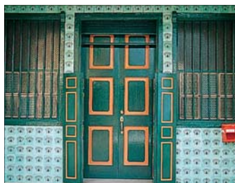
Tiled shophouse façade at Ann Siang Hill
