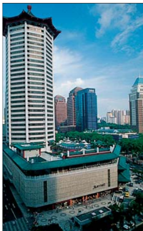
Singapore Marriott, located at a busy intersection on Orchard Road
