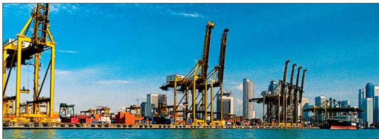
Computerized container facilities at the port
