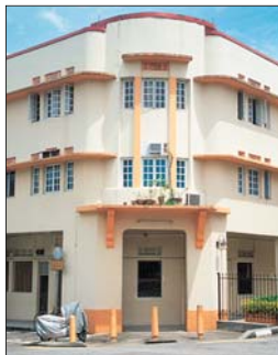
1930s Art Deco apartment block in Tiong Bahru housing estate
