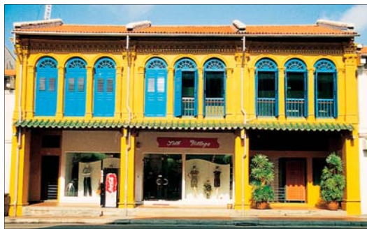
Restored double-storey shophouses along Duxton Road
