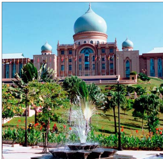
Palace of Justice, Putrajaya, with its distinctive Islamic-style architecture
