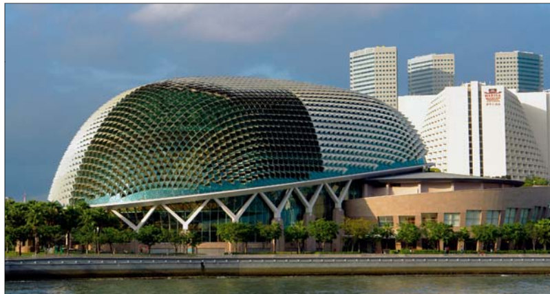
The massive riverside complex of Esplanade – Theaters on the Bay
