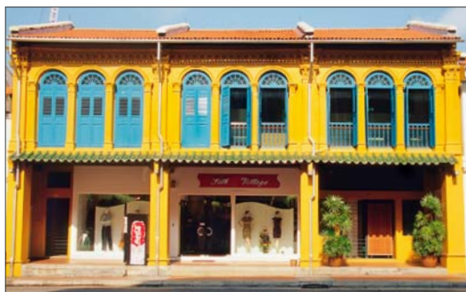
Restored double-story shophouses along Duxton Road
