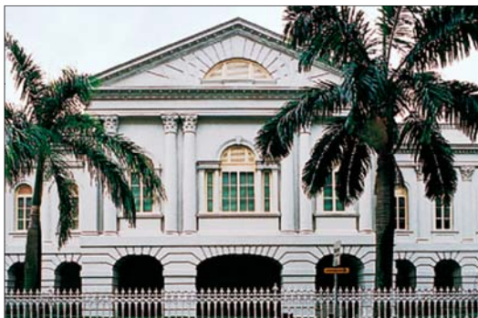
The Neo-Palladian façade of the Old Parliament House
