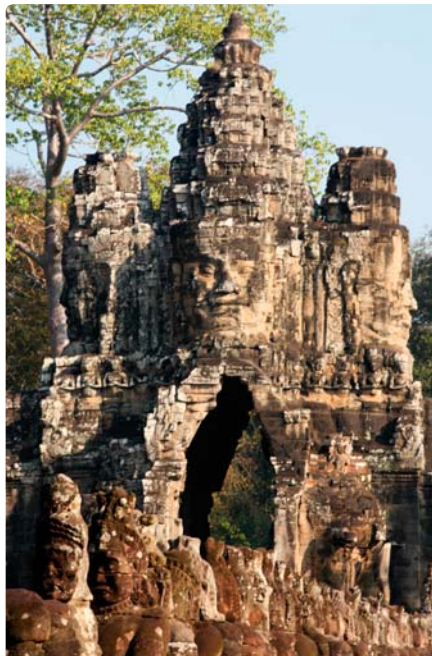
▼ South Gate, Angkor Thom
