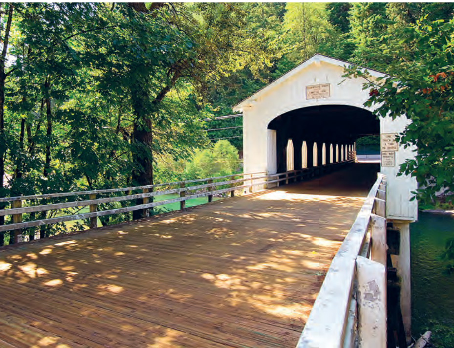
Goodpasture Bridge Oregon's second-longest wooden bridge
