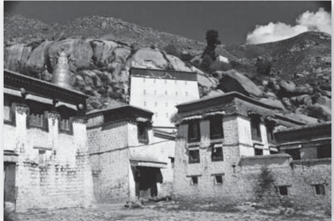
A corner of Ganden monastery near Lhasa, showing typical Tibetan architecture with its sloping walls, increasing window sizes and flat roofs. Behind is the huge wall on which painted scrolls (the Tanka) are hung during Buddhist festivals.
