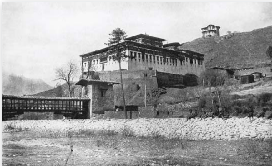
White's photograph of Paro dzong (1905) illustrates the defensive complex that was to be found at many of the Shabdrung's dzongs. Above the fortress monastery is the ta dzong with a fortified bridge in the foreground. The dzong is surrounded by an outer enceinte.
