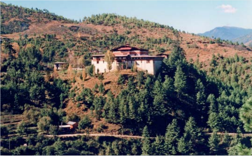
Simtokha dzong was the first of Ngawang Namgyal's (the Shabdrung) fortress monasteries combining the functions of monastery, administrative centre and fortress. Building commenced in 1629.
