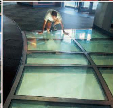
◀ Glass Floor The ground is more than 1,122 ft (342 m) below this thick layer of re-inforced glass, made from 256 sq ft (24 sq m) of solid glass that is five times stronger than the weight-bearing standard for commercial floors.
