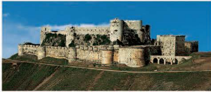
Tower of the King's Daughter > The northern face of this tower has a large projecting gallery from which rocks could be hurled if the outer wall was breached. At ground level, the tower is decorated with three blind arches.
