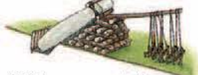
With levers supported by timber packing, the stone was gradually raised by 200 men.
