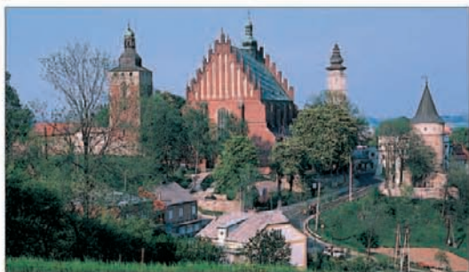
View of the Parish Church of Corpus Christi in Biecz
