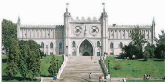
Neo-Gothic façade of Lublin Castle
