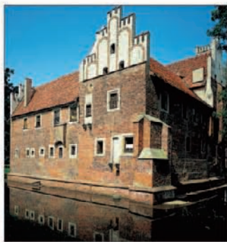
Moated Renaissance manor house in Wojnowice
