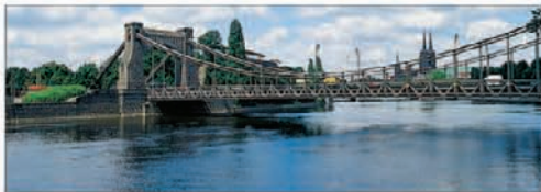
Grunwaldzki Suspension Bridge
