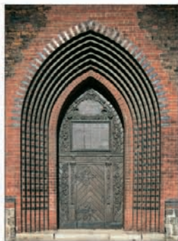
Portal of the Cathedral of St James
