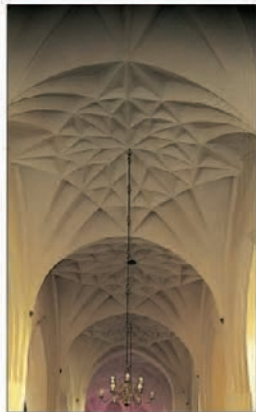
Crystalline vaulting in the Church of St George in Kętrzyn
