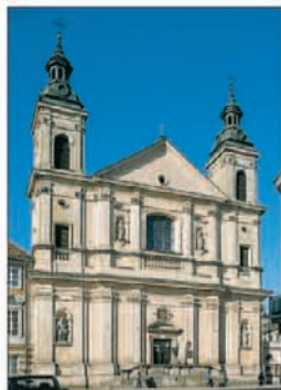
Church of the Holy Spirit, facing down Ulica Mostowa
