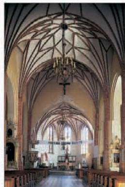
Star vaulting over the nave of Łomża Cathedral
