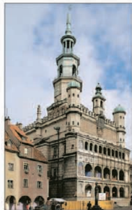
The Renaissance town hall, with its three tiers of loggias
