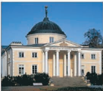
Lubostroń Palace viewed from the courtyard
