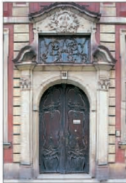
The Rococo doorway of Uphagen House
