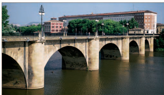
The stone Puente de Piedra, spanning the Ebro river in Logroño
