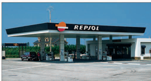
A petrol station belonging to the Repsol chain
