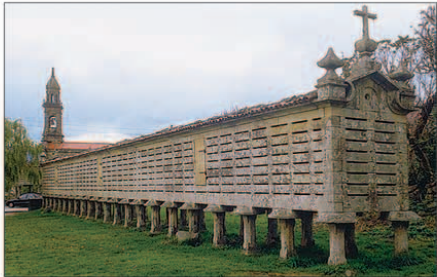
This hórreo (granary) in Carnota, dating from 1760 and extending 35 m (126 ft), is one of the largest in Galicia. Hórreos were built on stone legs to protect the grain from damp and pests. The cross is a decorative motif.
