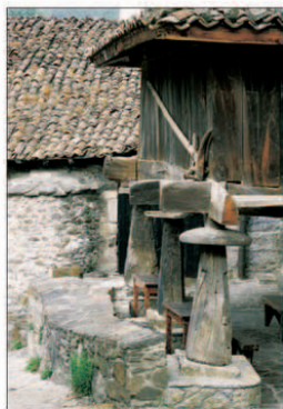
A typical red-roofed wooden hórreo (granary) in Bárzana
