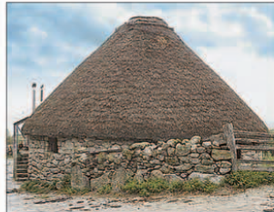
Pallozas are among the oldest structures built in Europe. Dating from Celtic times, these houses have thick walls and thatched roofs. The inhabitants used to divide the space into living quarters, animal stables and a food store.
