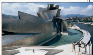
Rare materials, such as titanium, were used in the construction of the futuristic Museo Guggenheim in Bilbao (see pp124–5) by Frank Gehry.
