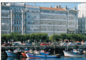
Houses with impressive glass balconies in the port area of A Coruña
