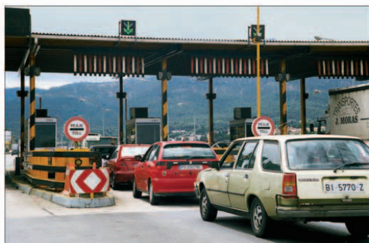
The toll-booth barrier at the entrance to a motorway
