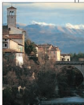
The bridge at Cividale del Friuli
