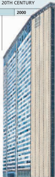
The Pirelli building in Milan, designed by Ponti and Nervi (late 1950s), is a great example of modern Italian architecture (see p185).
