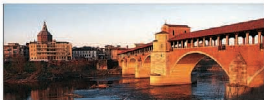
The partly Renaissance Ponte Coperto, straddling the Ticino River at Pavia
