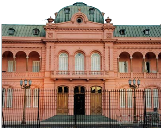
The striking neoclassical façade of the Casa Rosada
