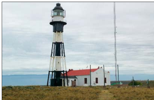
The lighthouse built by the Argentinian Navy at Cabo Vírgenes
