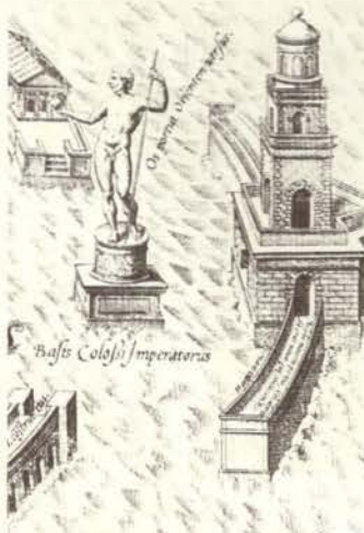
Towered docks at Rome's harbor, built by the emperor Claudius
