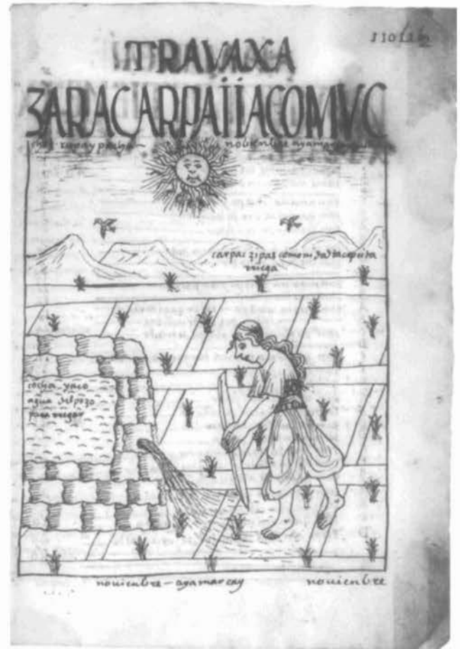
FIG. 6.10. THE ORGANIZATION OF ANDEAN LAND-HOLDINGS AS A GRID. In addition to radial and strip divisions of land, grids were also employed in Andean spatial organization. A grid of shallow ditches separates Inka agricultural plots during the planting and growing seasons in this drawing by Felipe Guamán Poma de Ayala. Springs, reservoirs, ditches, and canals functioned as social and territorial boundary markers in traditional Andean society.
