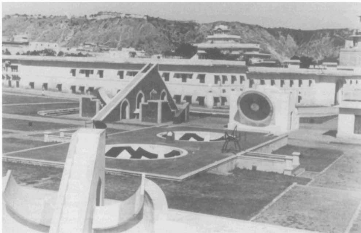
FIG. 16.23. JAIPUR OBSERVATORY. This photograph, taken from atop the Saṃraṭ Yantra within the Jaipur observatory built by Jai Singh, shows several of its giant masonry instruments. The Saṃraṭ Yantra, a triangular gnomon, has a height of nearly 90 feet, above the ground and a base of 147 feet. The corresponding instrument at Delhi is substantially smaller (60 feet, 4 inches high). The two complementary concave hemispheres of the Jai Prakāṣa (17 feet, 10 inches in diameter) appear in the
