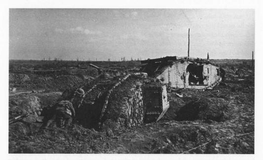
Two Mark IV tanks. A camouflaged male stuck in a shell hole and a damaged female ahead of it, with dead or wounded soldiers.
