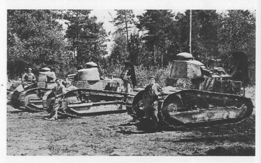
A group of Renaults with their crews preparing for action. All are equipped with 37 mm cannon, but whereas the centre tank has a cast turret the other two are of the built-up type.
