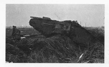
A Mark II male tank crossing a shallow trench on its way forward. The piece of wood at the front is a torpedo spud attached to the track. It was used to help a tank unditch itself in muddy conditions.
