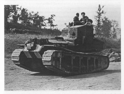
A Whippet going forward, with two of its crew taking the air. Extra petrol cans are strapped on the front.
