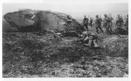
Tank No. 599, a Mark II female, moving forward with infantry. Compare the Lewis guns in the sponson with the heavy Vickers guns, in their armoured jackets, on the Mark I female tanks in Chapter 1.
