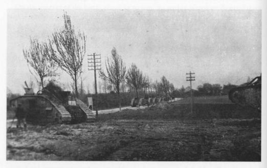
Mark V tanks trekking from a railhead. The new engine and transmission made these tanks much less tiring to drive over long distances than the old Mark IVs.
