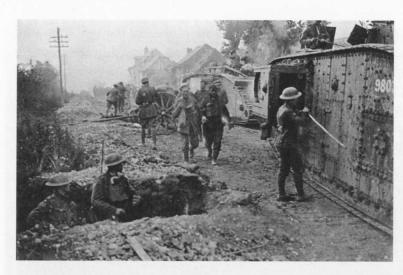
A Mark IV supply tank leads a Mark V\* female tank through a captured village.
