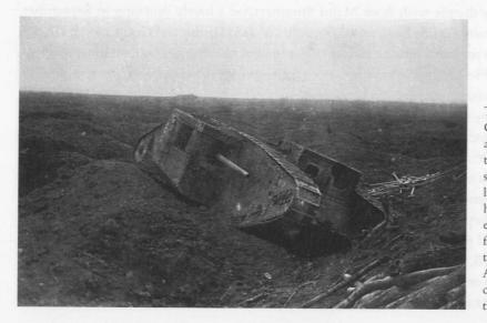
The male tank C3, having taken a direct hit on the commander's side of the cab, lies in a shell hole. There is evidence of a failed attempt to dig it out. Another tank can be seen in the distance.
