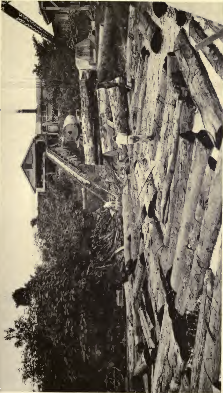
FIG. 13. Nanay mills, near Iquitos, showing the log haul-up.
