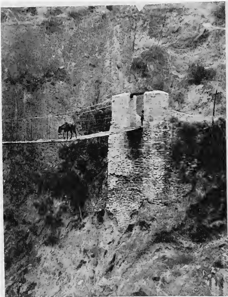
BRIDGE OVER GORGE OF RIO DE PAMPAS See p. 178
